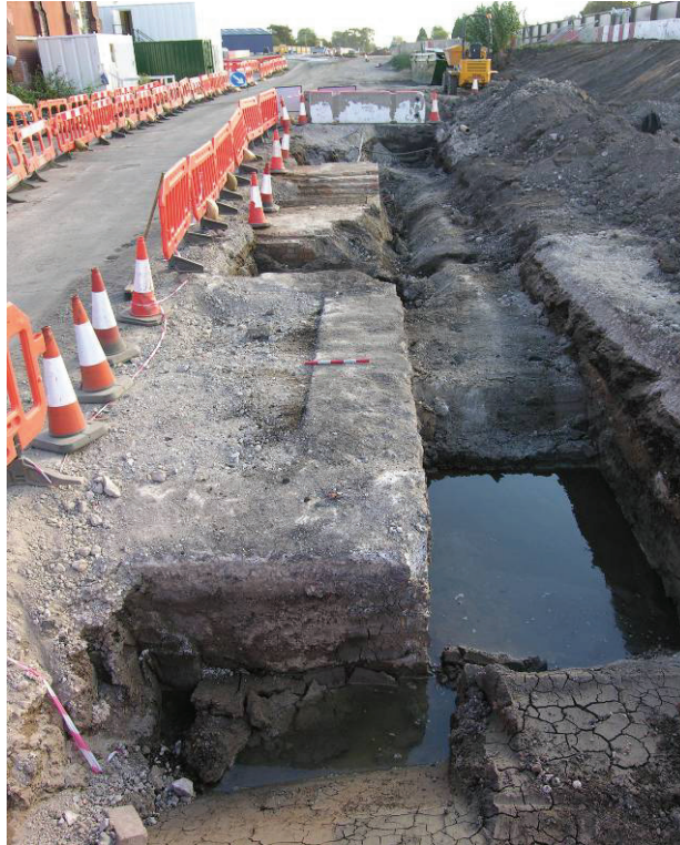
Photo 36. The concrete structure, or cooling tower, looking east with the brick chimney base in the background
