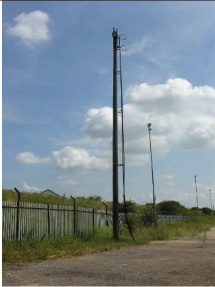
Photo 16. Item 7, The laddered telegraph pole, looking east.
