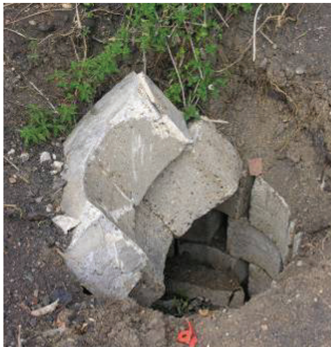
Photo 26. The remains of the air vent to the west of the shelter
