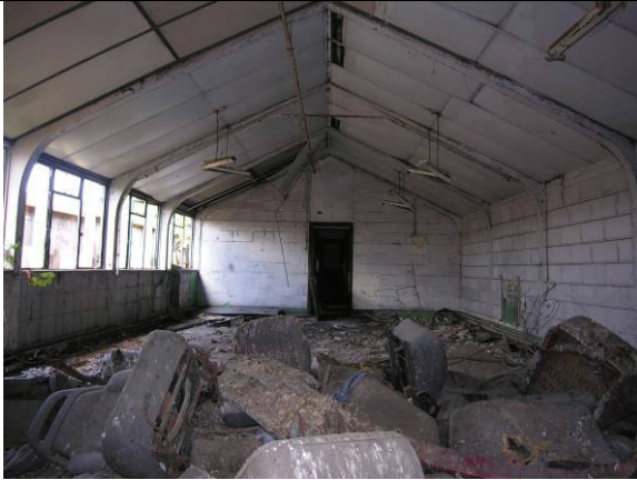
Photo 12. The interior of the southern annexe of building item 4, looking north.
