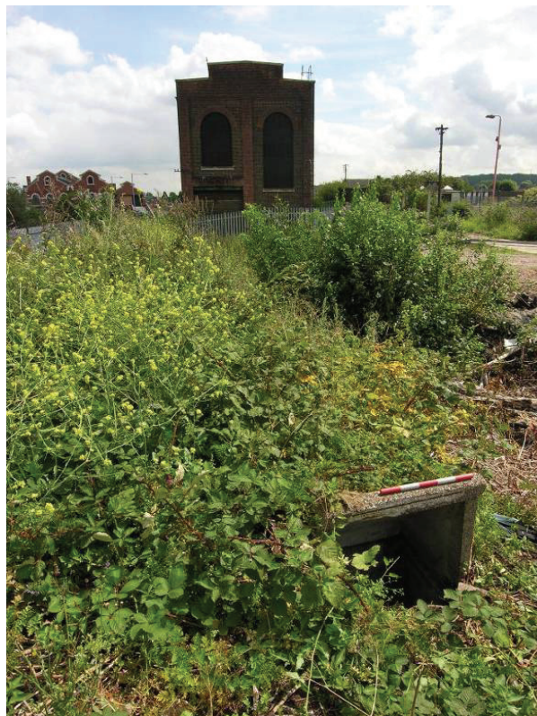
Photo 29 The entrance to the escape hatch in the foreground, the electricity substation, Item 3 is in the background.
