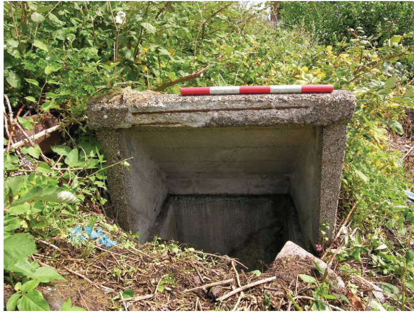
Photo 30. The concrete escape hatch looking east.
