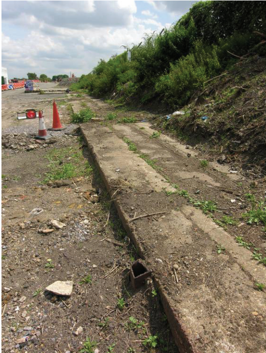
Photo 2. The concrete track bed looking south east.
