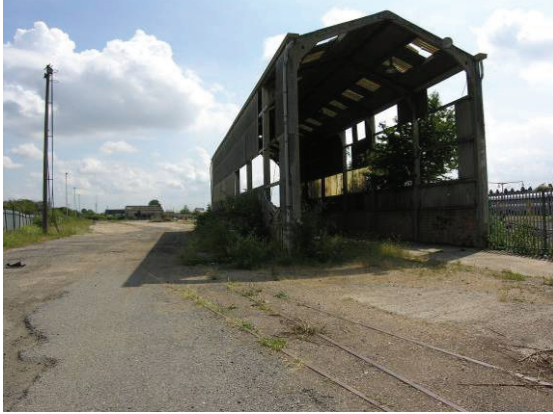
Photo 18. The railway tracks looking towards the south-east showing their position in relation to the engine shed (Item 6).
