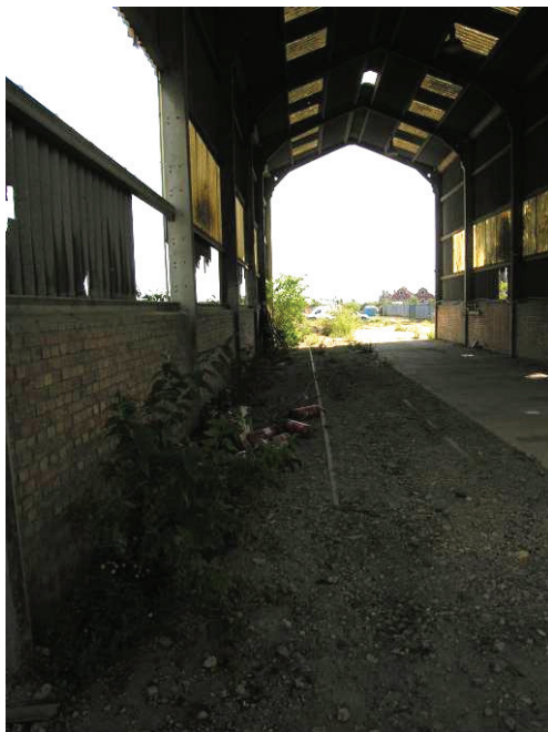
Photo 15. The interior of the structure looking east.
