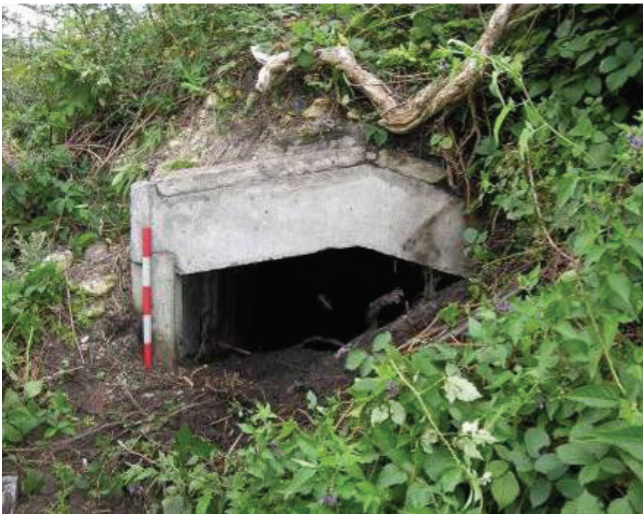
Photo 27. A view of the entrance to shelter 2 at its eastern end looking west
