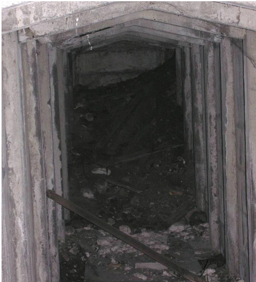
Photo 31. The internal view towards the western end of the shelter and the concrete wall behind the collapse of earth
