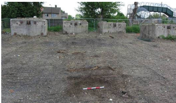
Photo 5. The group of concrete buffer blocks at the far eastern end of Worksite east, looking east.
