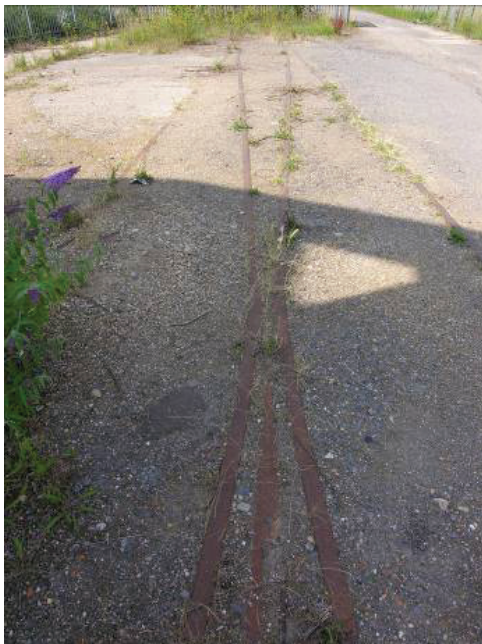
Item 8 Series of disused railway lines at west end of old Goods yard.
