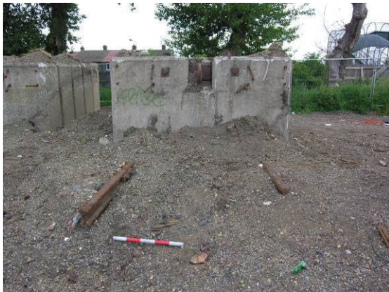
Photo 7. The former tracks visible running beneath the southernmost block, looking east.
