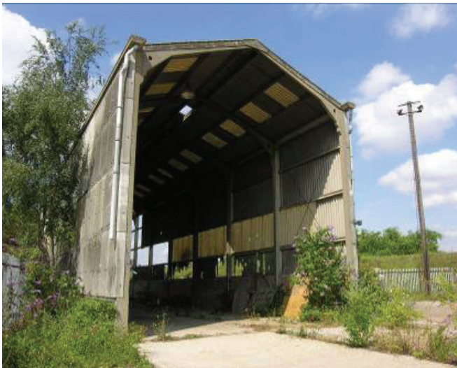
Photo 13. Building item 6, the train shed, looking north west.
