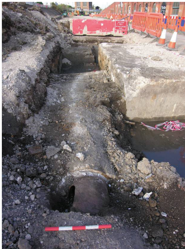
Photo 37. The exposed section of the pipe emanating from the former cooling tower
