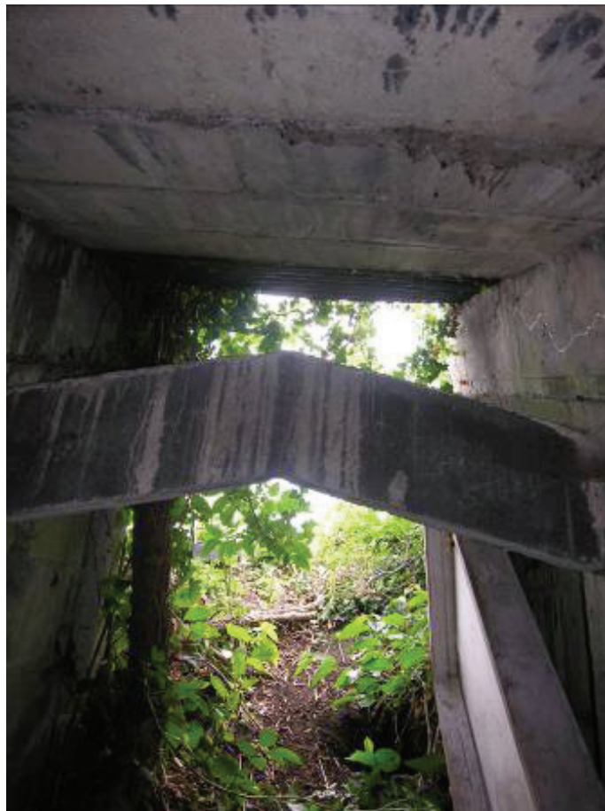
Photo 24. The entrance of Shelter 1 from within, looking south
