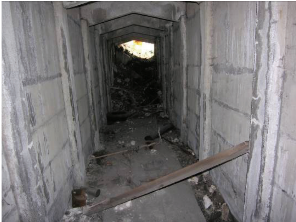
Photo 28 An internal view of shelter 2 looking east towards the present entrance
