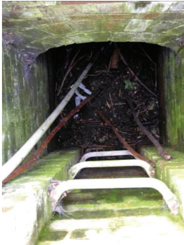
Photo 25. The escape shaft to the south of the shelter, with the brick tunnel running to the west
