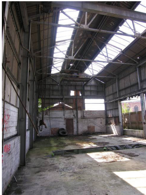
Photo 11. The interior of building item 4, looking south.
