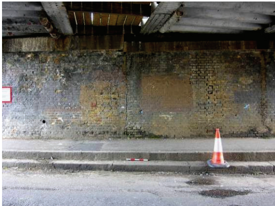
Photo 22. The kerbstones beneath the railway bridge on White Hart Road, looking east. Note the two separate builds visible in the fabric of the bridge
