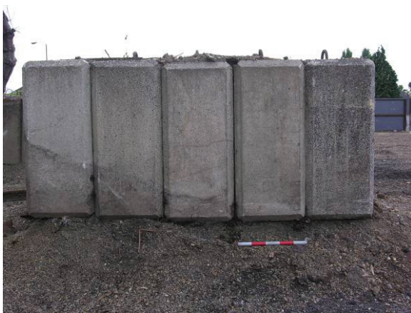
Photo 6. The side view of one of the blocks showing its composition from five separate blocks, looking south.
