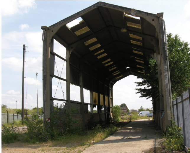
Photo 14. The western end of the building looking east.
