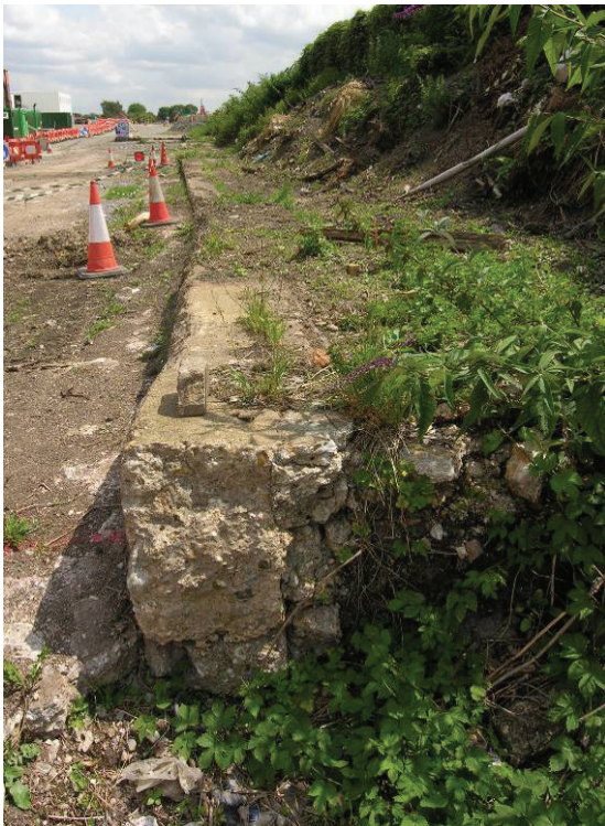
Photo 3. The truncated western end of the concrete track bed.
