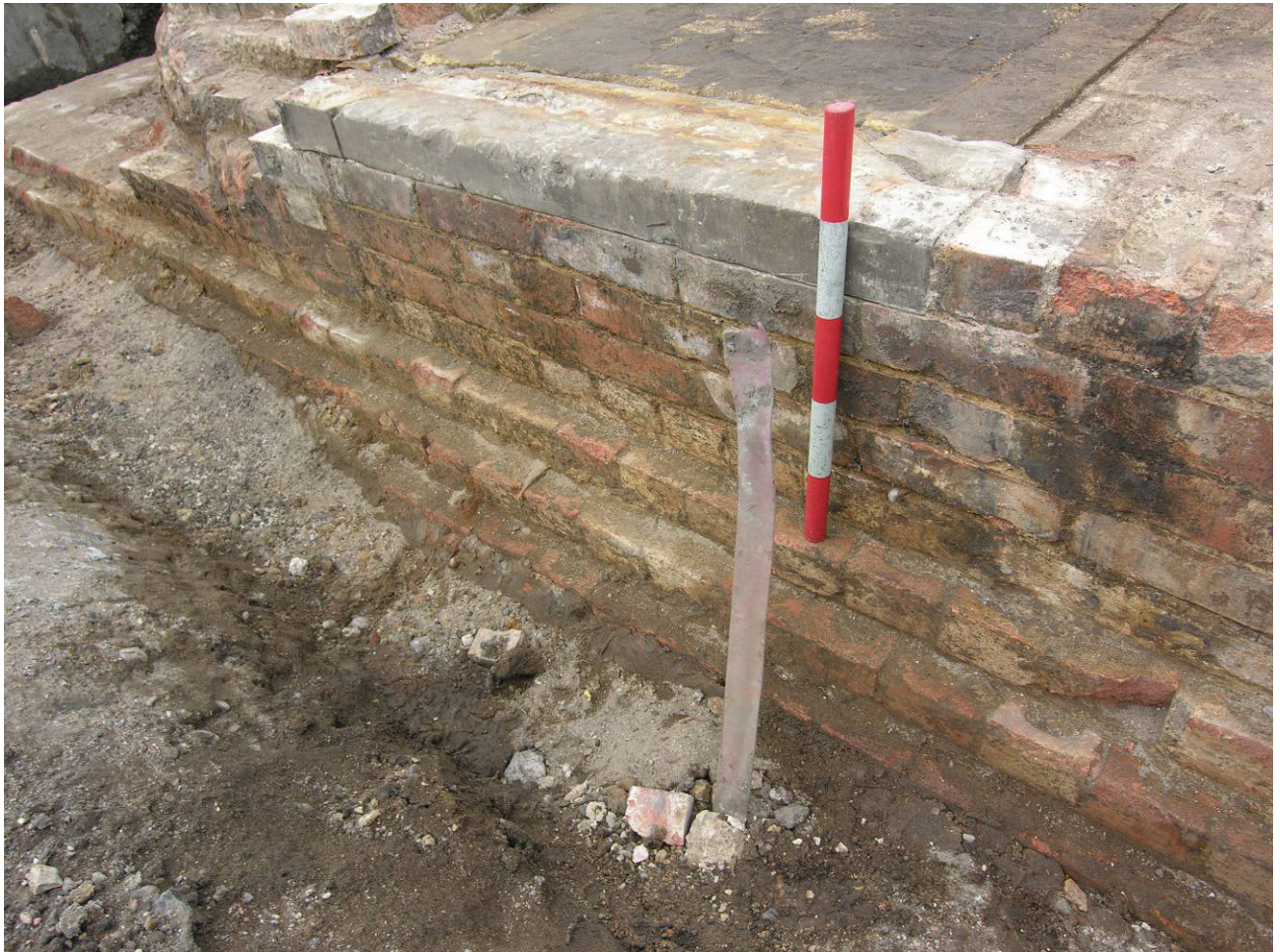
Photo 35. The copper lightning conductor and the stone sill on the southern side of the brick structure
