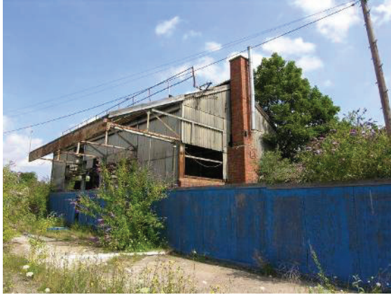
Photo 10. Building item 4, looking north east.
