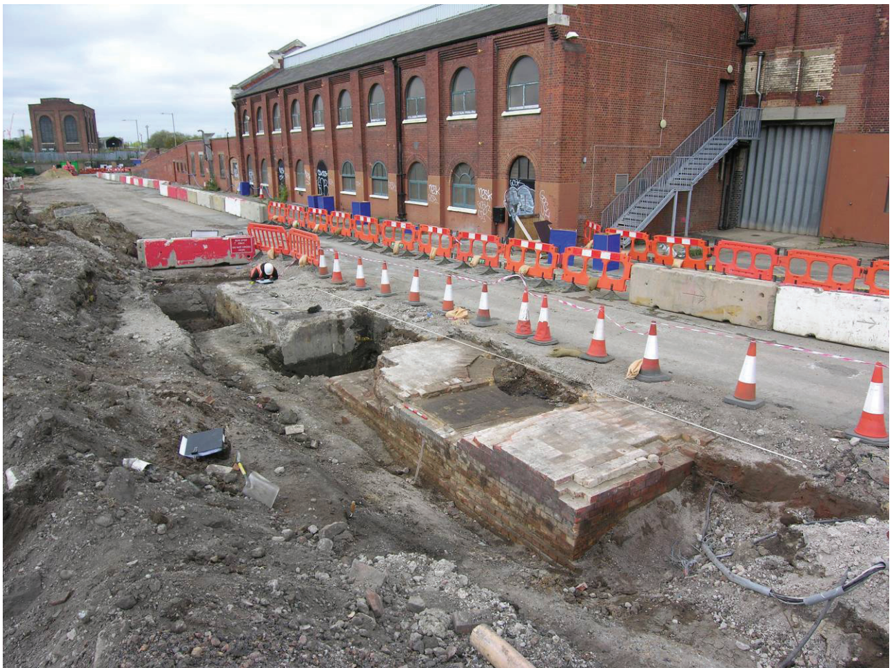
Photo 32. The excavations looking north east and the location of the recorded features in relation to the Listed Depot building
