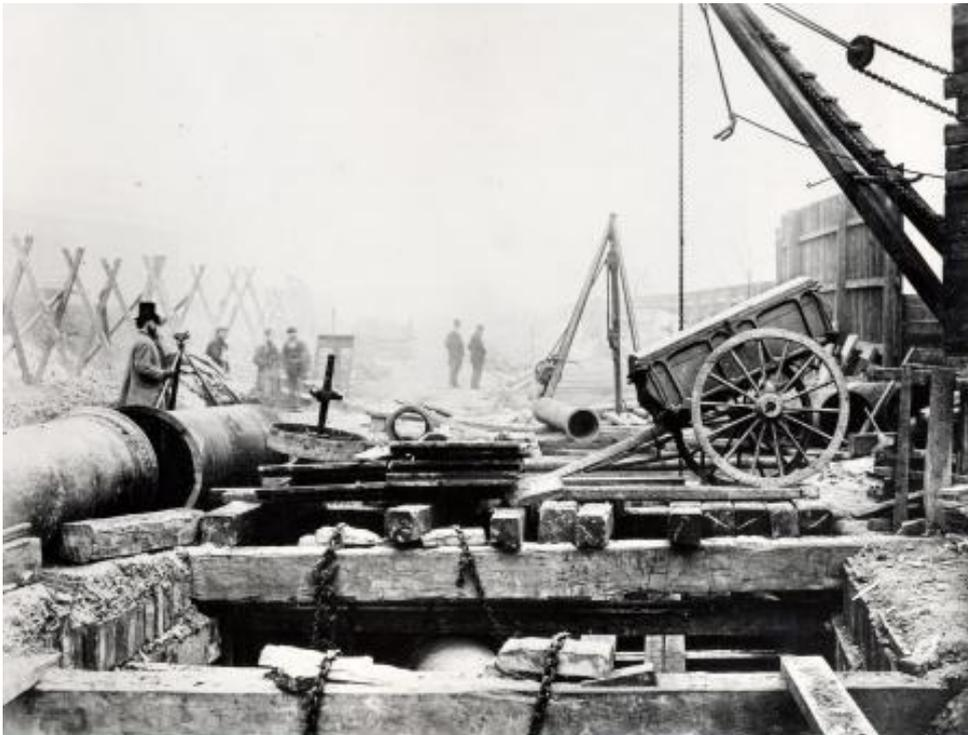
Figure 4. Photograph of the cut and cover construction of the Metropolitan Line extension to Kensington c. 1867 (Collection of the London Transport Museum)
