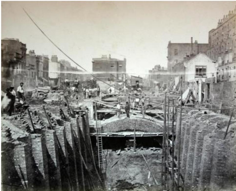
Figure 3. Photograph of the cut and cover construction of the Metropolitan Line at Praed St, Paddington c.1866 (Collection of the London Transport Museum)
