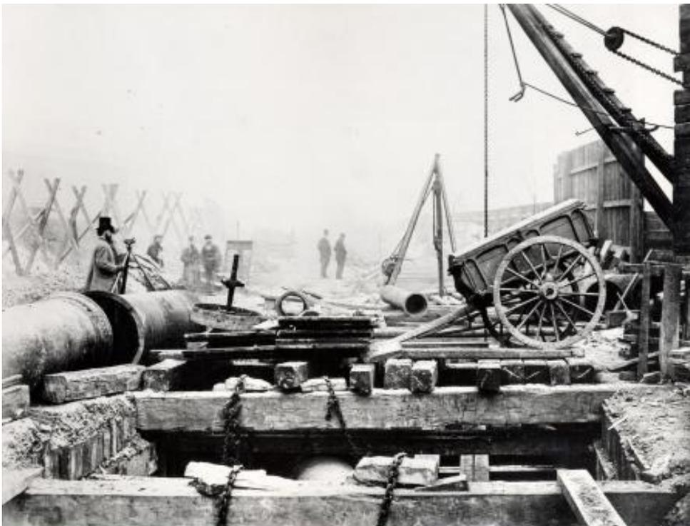
Figure 4. Photograph of the cut and cover construction of the Metropolitan Line extension to Kensington c. 1867 (Collection of the London Transport Museum)
