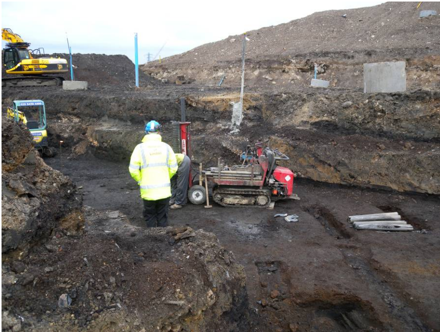
Photo 8: Trench 2 with terrier rig in operation, looking north-west
