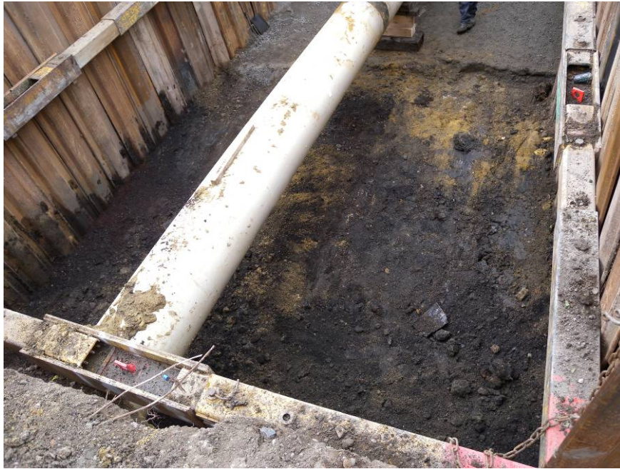
Photo 14: Base of eastern stopple pit, looking north-east
