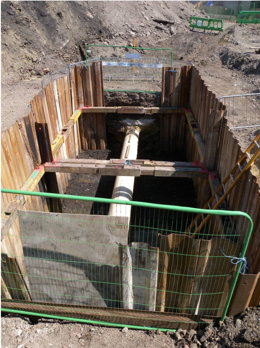
Photo 13: Eastern stopple pit, looking east
