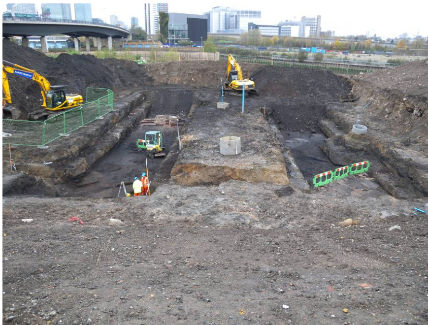
Photo 4: Trench 2 (left), with timber baseplates with concrete [32] & [33] and timber sleepers (front) and brick structure [31] (rear), looking west
