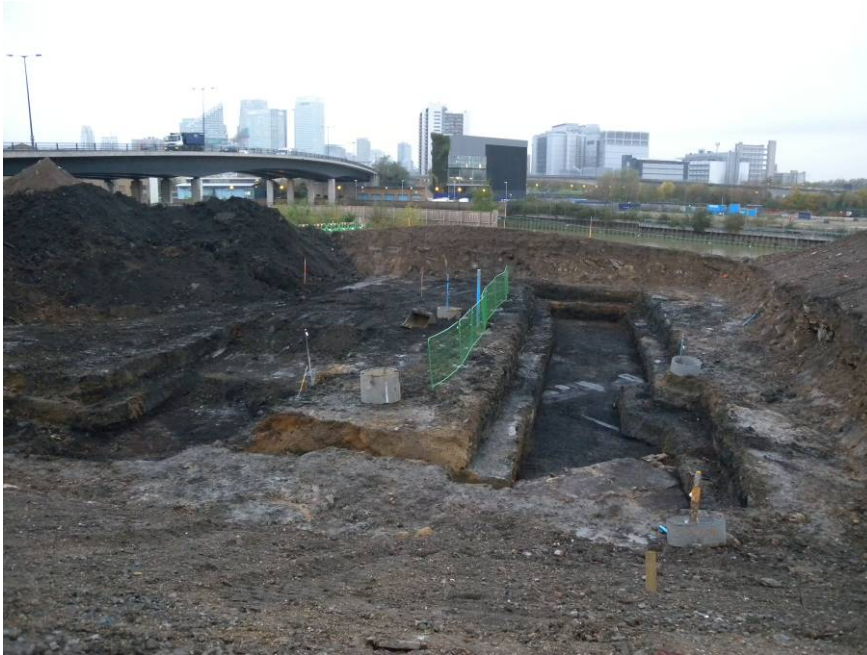
Photo 1: Trench 1 (right) with Structures [12] and [13] (front), timbers [16] & [15] and concrete pads [14] (centre), looking west
