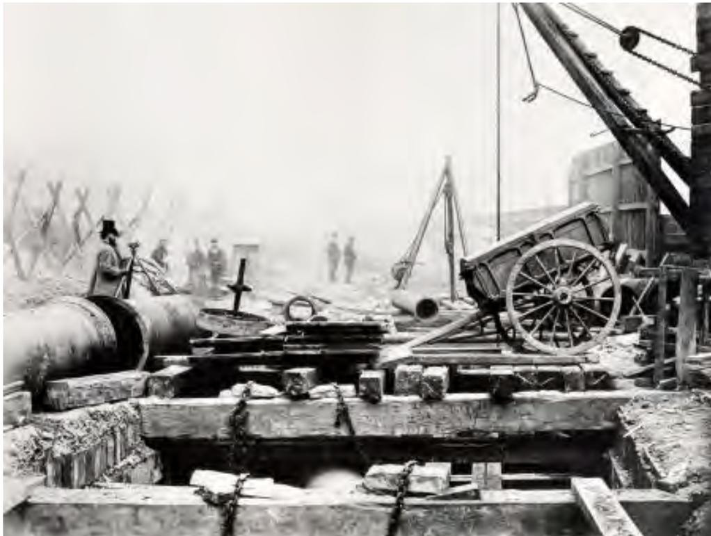
**Figure 2. Photograph of the cut and cover construction of the Metropolitan Line extension to Kensington c. 1867 (Collection of the London Transport Museum)**
