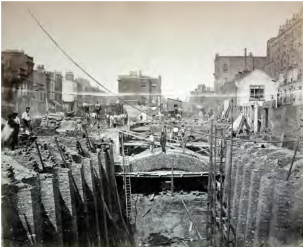
**Figure 1. Photograph of the cut and cover construction of the Metropolitan Line at Praed St, Paddington c.1866 (Collection of the London Transport Museum)**
