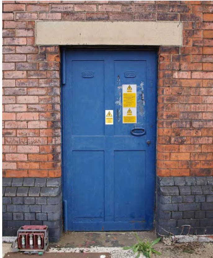
Plate 53. Steel door at west end of Substation B2 (26)
