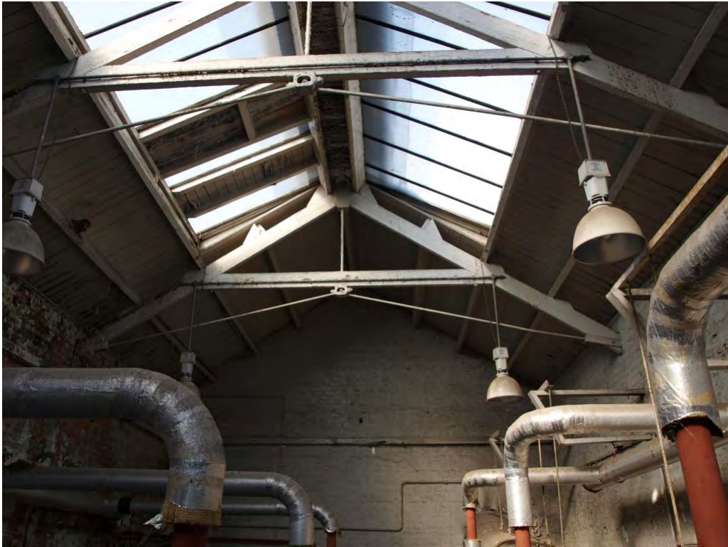
Plate 45. Composite roof truss, south side of Factory Boiler House (former Carpenters' and Coppersmiths' Shop) (15c)
