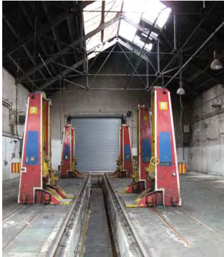
Plate 17. Interior of the Factory Lifting Bay (15b), looking west.
