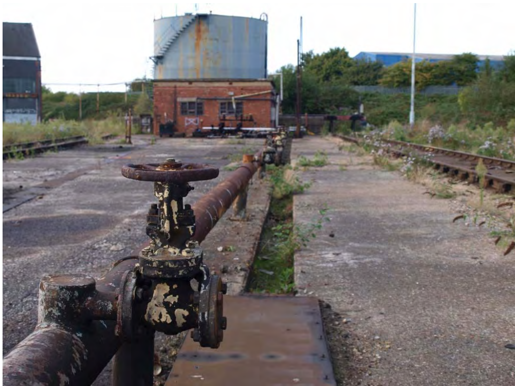
Plate 56. Heavy oil/diesel pipe and valves, Oil/Diesel delivery area (32)
