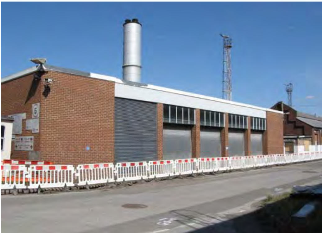
Plate 28. Pullman Shed Boiler House (21) looking north-east.
