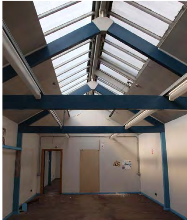
Plate 61. Composite roof trusses, Amenities Building, first floor (17a)
