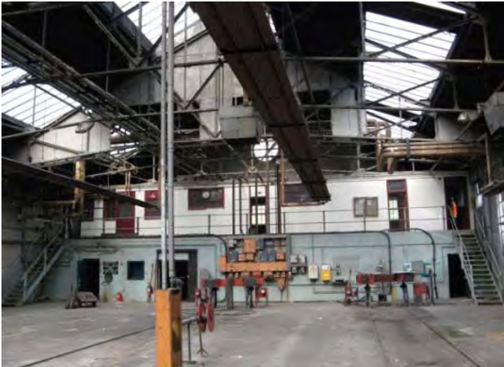
Plate 33. Original offices at west end of Pullman Shed (22).
