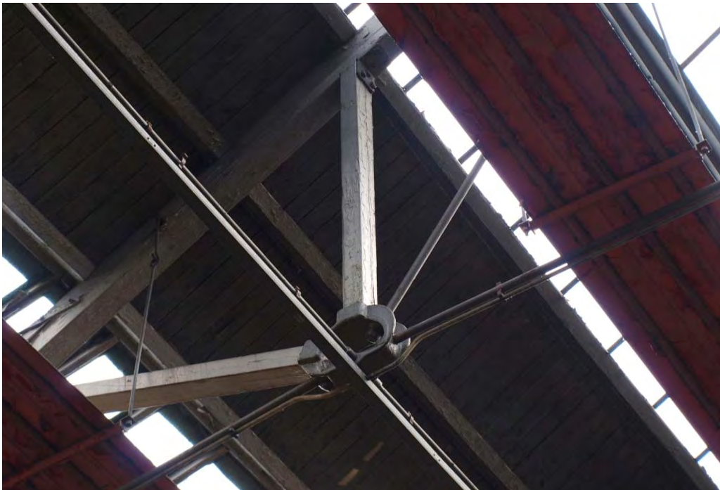
Plate 42. Composite roof truss, Factory former Lifting Shop (15a): Detail of cast steel junction ring
