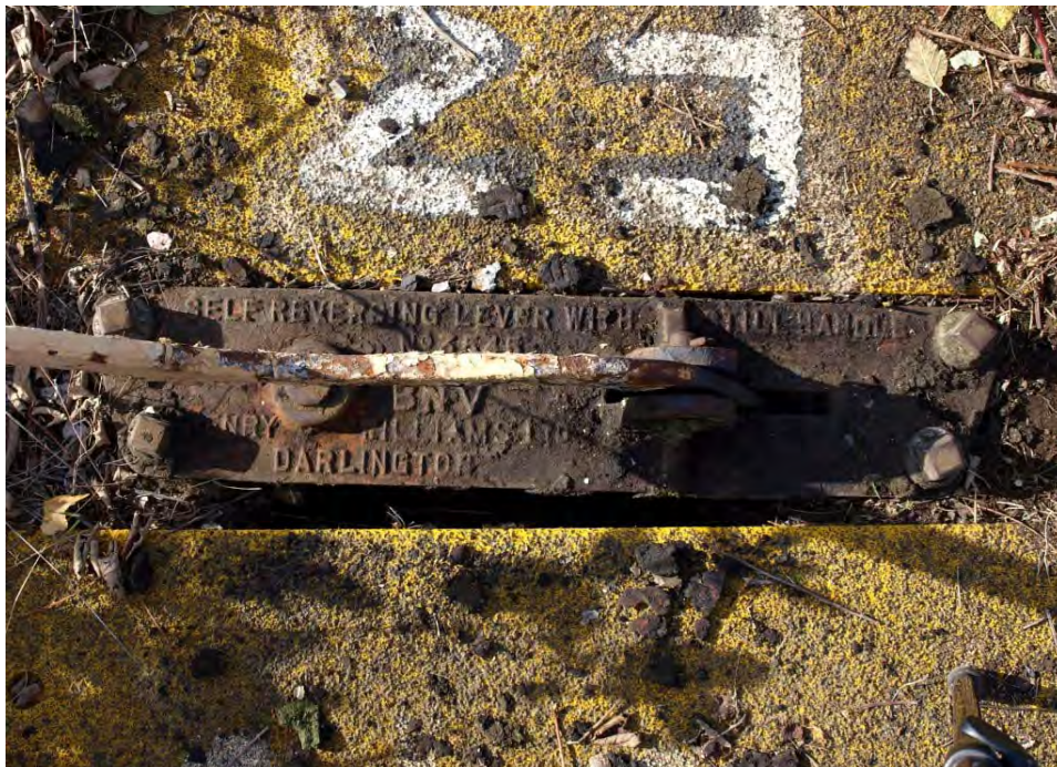
Plate 66. 'Self reversing' points lever baseplate, locomotive shunting yard, near Shunters' Cabin (1).
