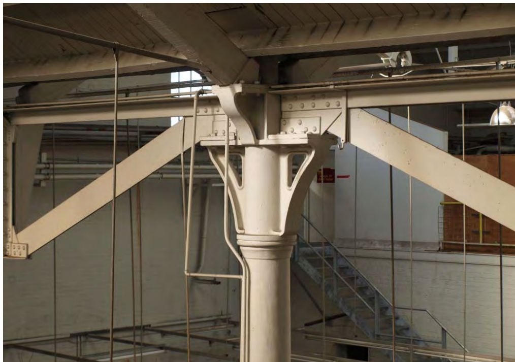
Plate 48. Detail of column capital, transverse beams and truss connection, Stores/Offices building (16a & 16b)
