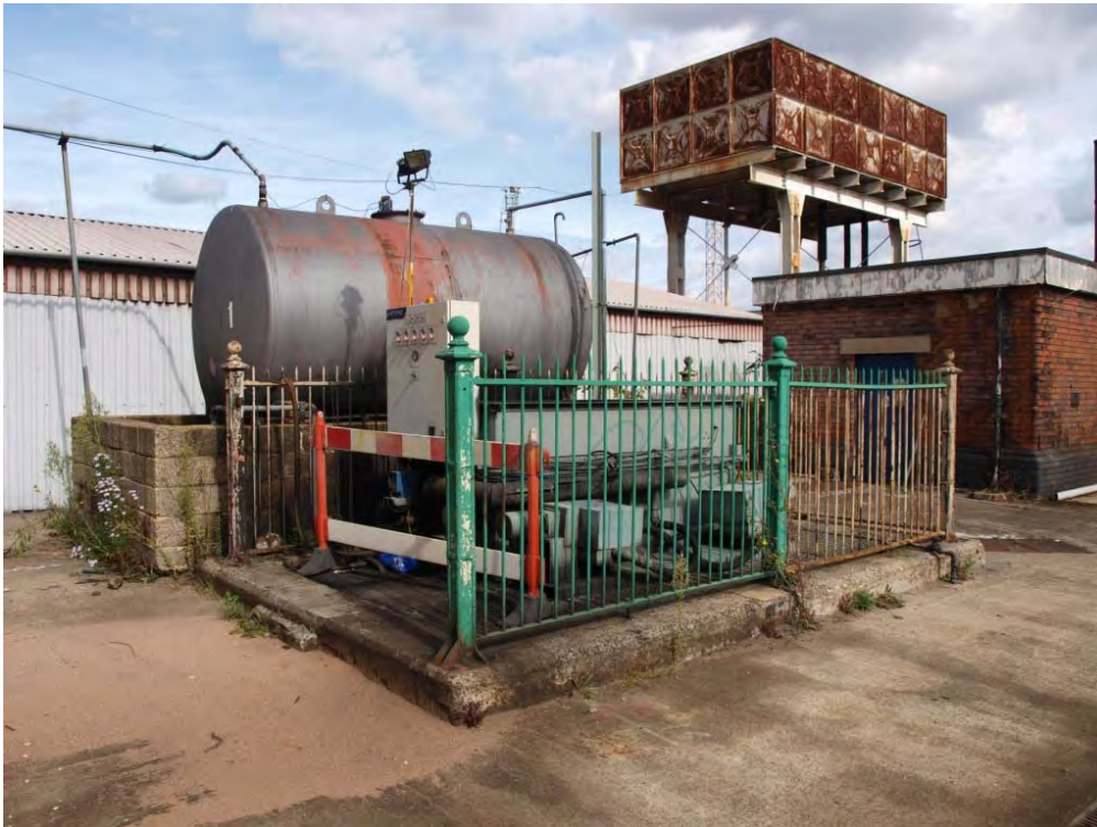
Plate 52. Cast iron railing, Sump/Oil Interceptor (24)
