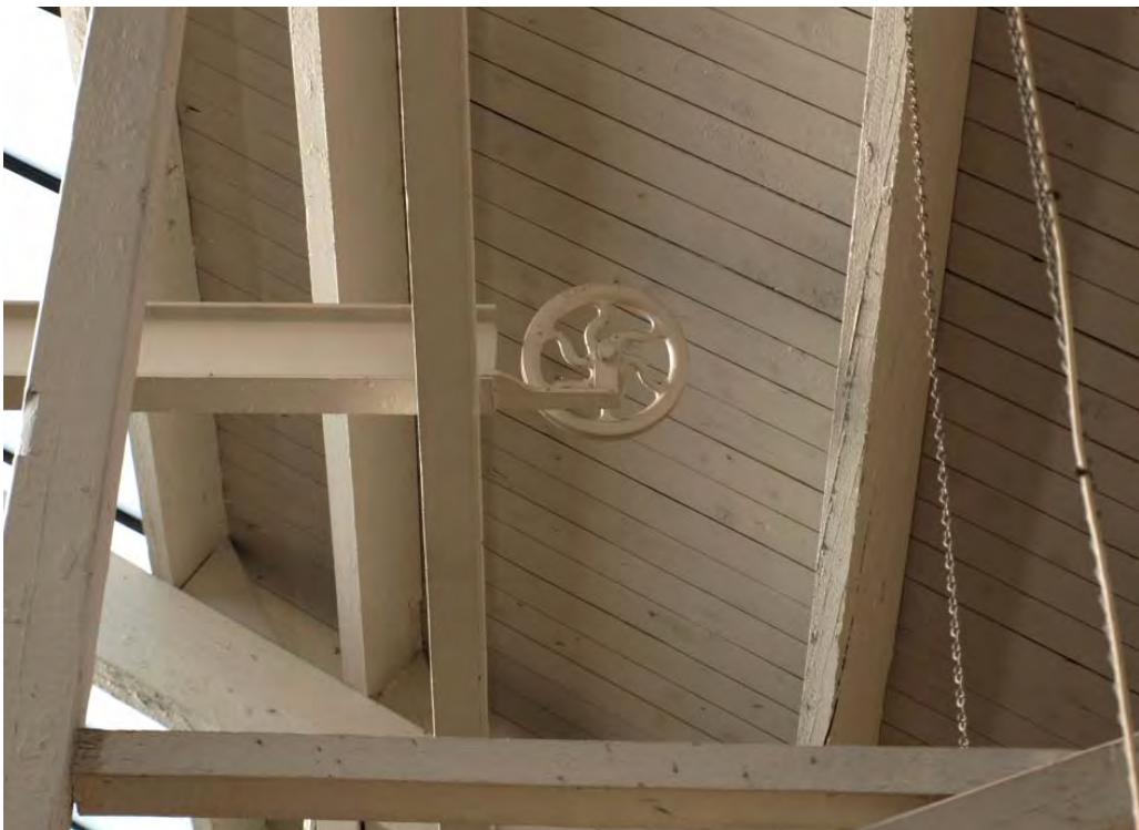
Plate 50. Detail of probable cast iron pulley wheel, Stores building (16a)
