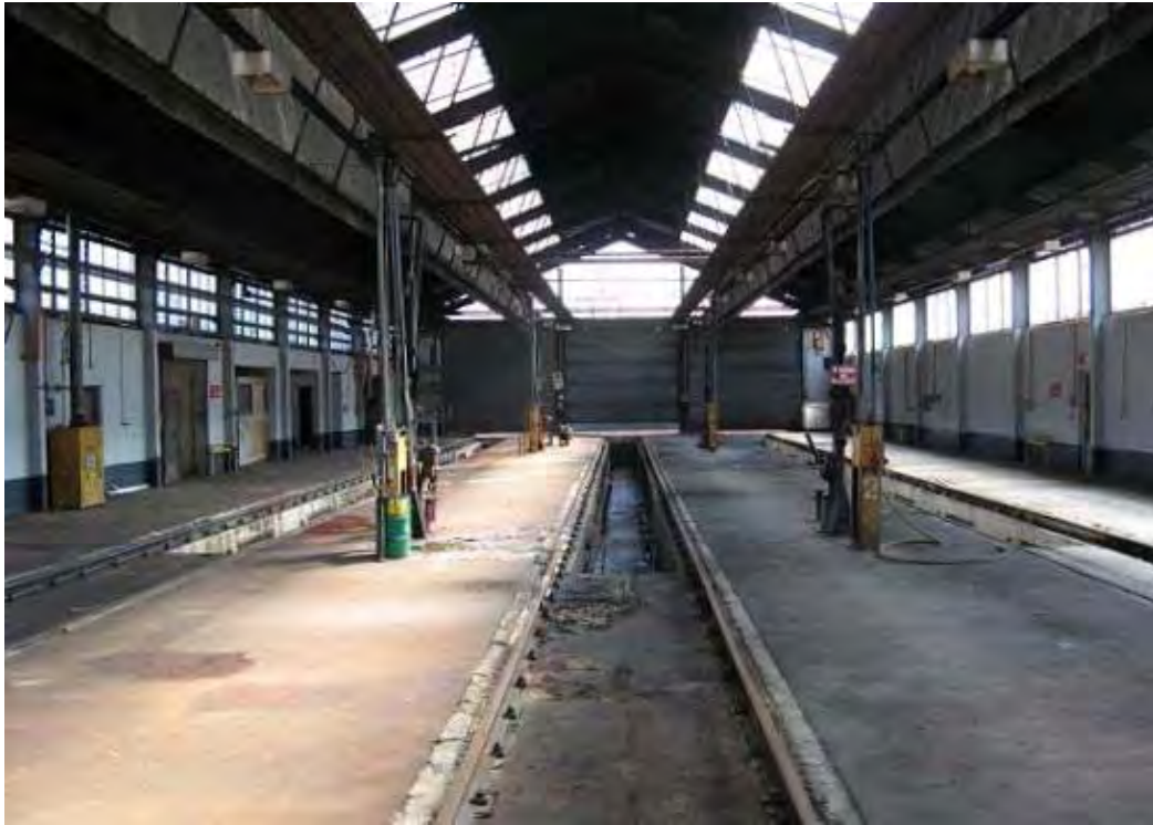
Plate 25. Interior of Diesel Refuelling and Maintenance Shed (19), looking east.
