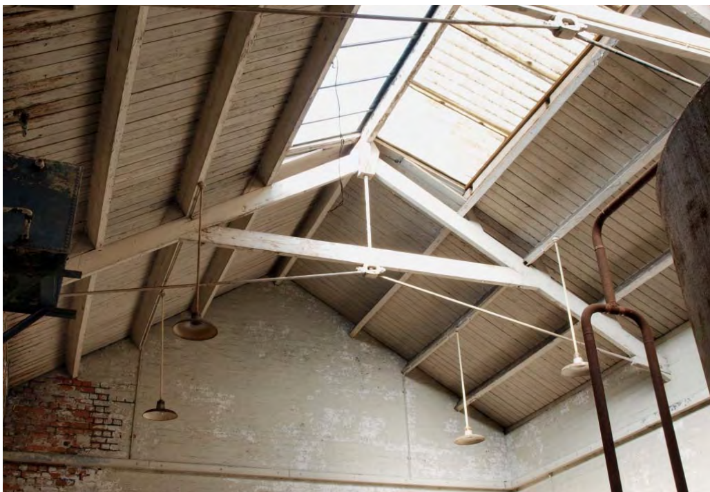
Plate 44. Composite roof truss, north side of Factory Boiler House (former Carpenters' and Coppersmiths' Shop) (15c)
