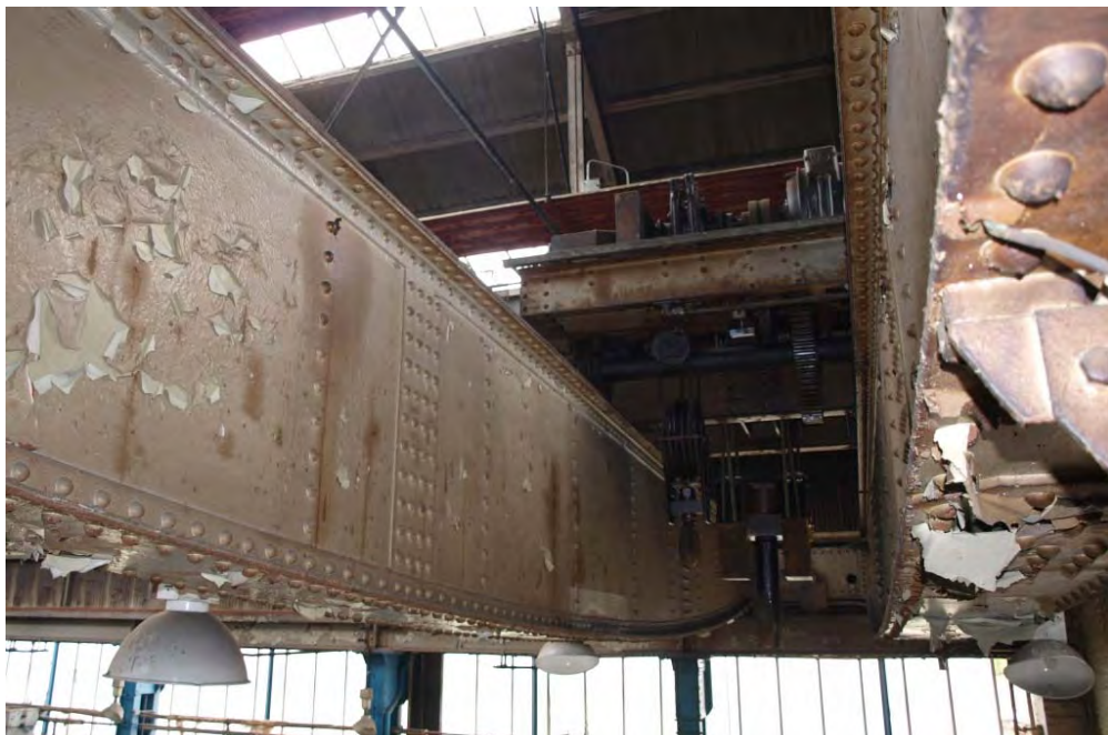
Plate 60. Detail of lifting gear of Heywood crane, Factory former Lifting Shop (15a)
