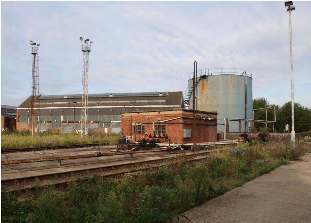
Plate 57. Diesel oil unloading jib, Diesel/Oil Tank and Pump House (6 & 53)
