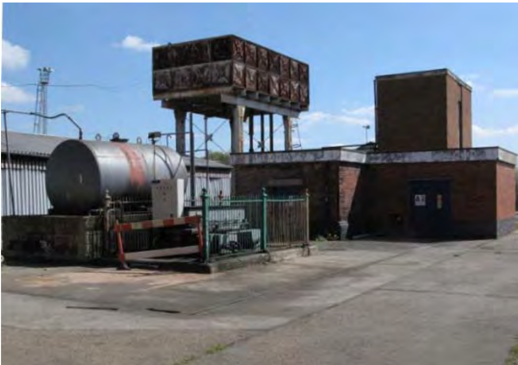
Plate 36. Sump/oil Interceptor (24), Bunded oil tank (54) and Sub Station B2 (26).
