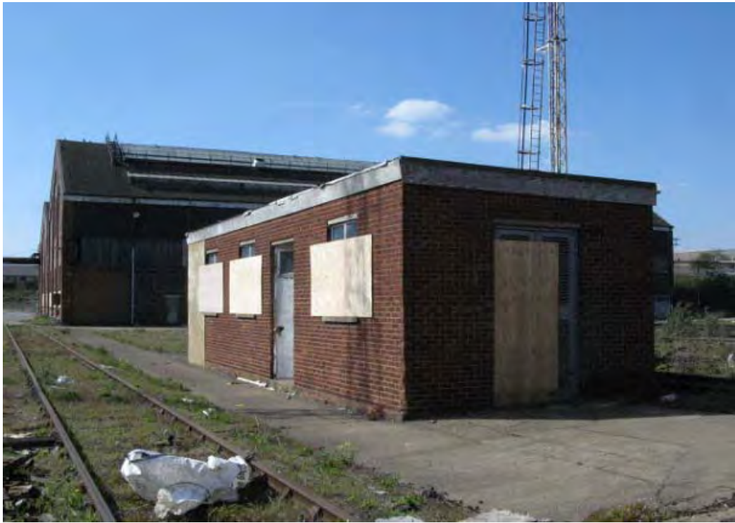
Plate 9. Steam Raising Plant (5), looking north-west.
