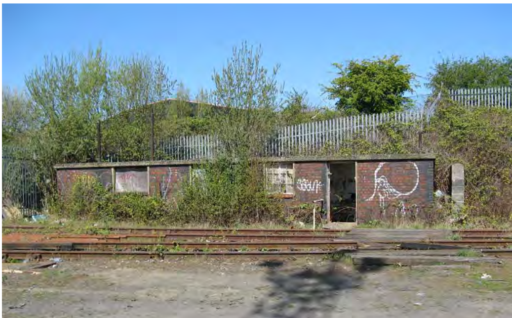
Plate 4. South elevation of 'Shunters Cabin' (1), former WWII air raid shelter.
