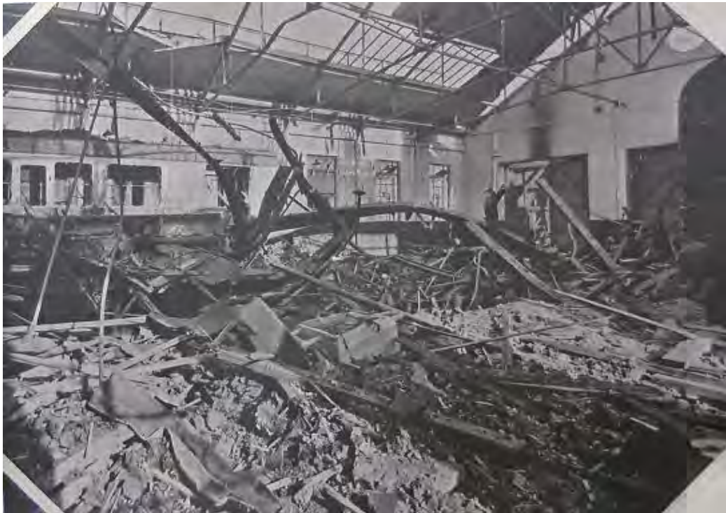
Plate 3. Pullman Shed (22) interior looking north east after air raid on 25/10/1940.
