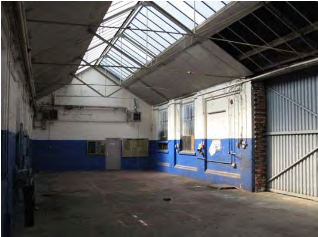
Plate 27. Mess Room/Sand Furnace (20) looking north-west, showing recessed panels on the once exterior face of the original 1905 Engine Shed wall which had been retained as the north wall of this building and enclosed when this building was extended.
