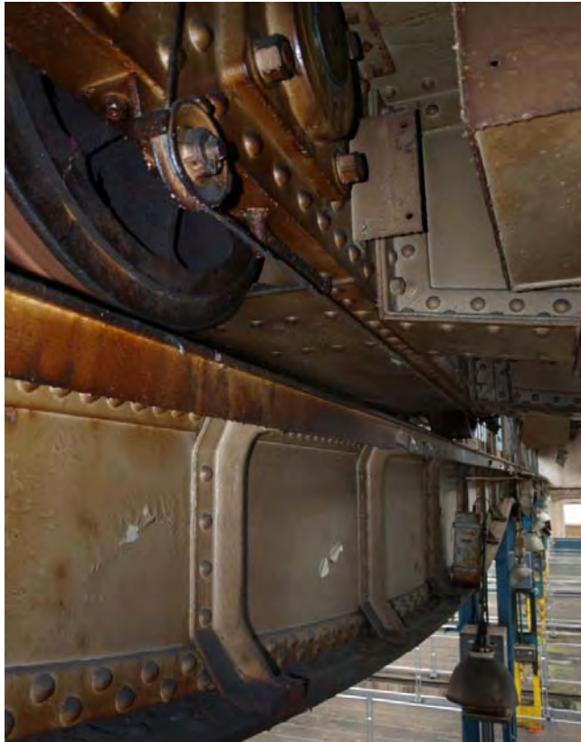
Plate 59. Detail of running wheel of Heywood crane on central 'fish belly' beam of Factory former Lifting Shop (15a)
