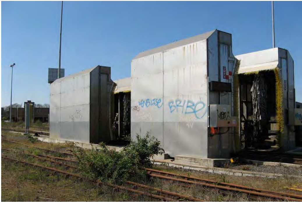
Plate 5. Carriage Washing Plant (3).
