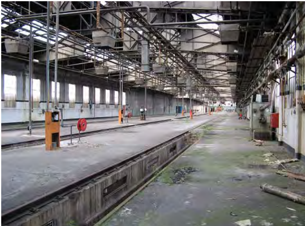
Plate 32. Interior of Pullman Shed (22) looking west.
