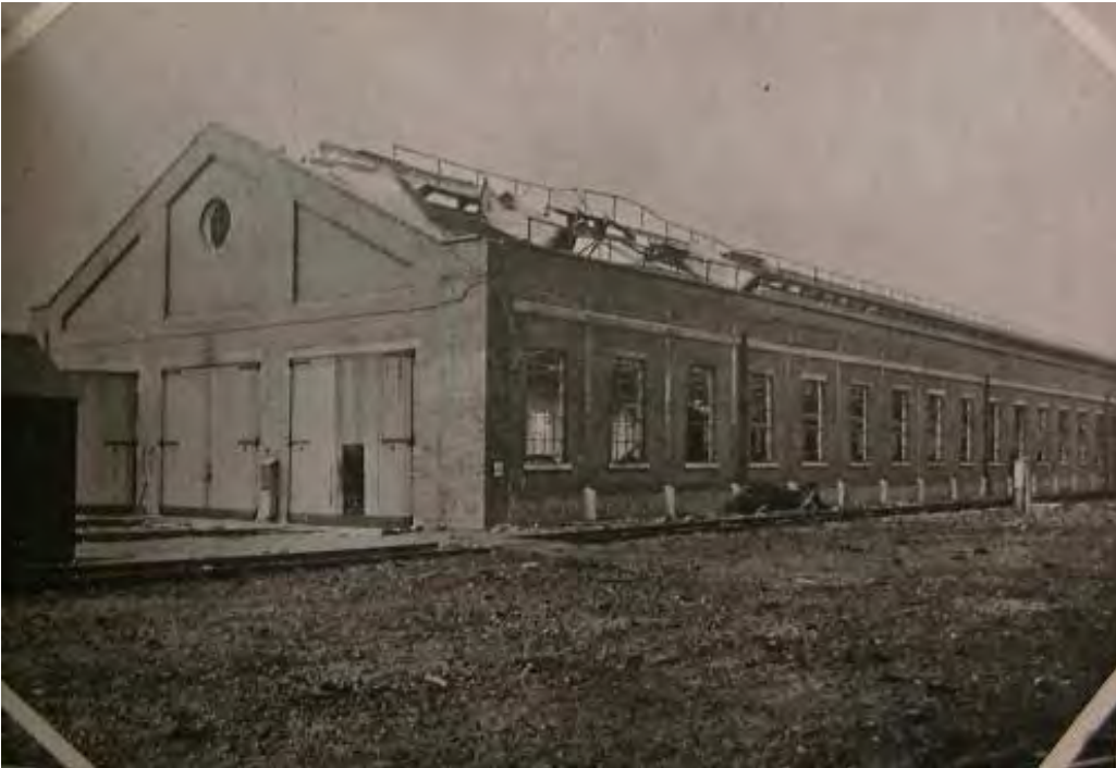
Plate 1. Pullman Shed (22) after air raid on 25/10/1940, showing damage to gable end and north wall.
