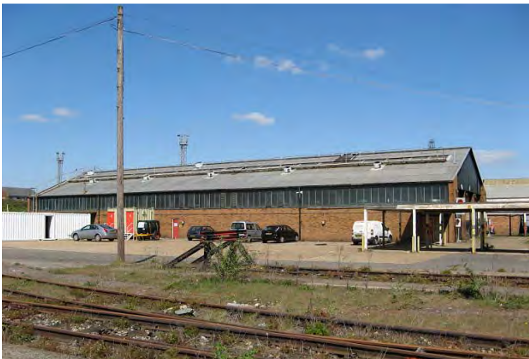
Plate 24. South elevation of Diesel Refuelling and Maintenance Shed (19).
