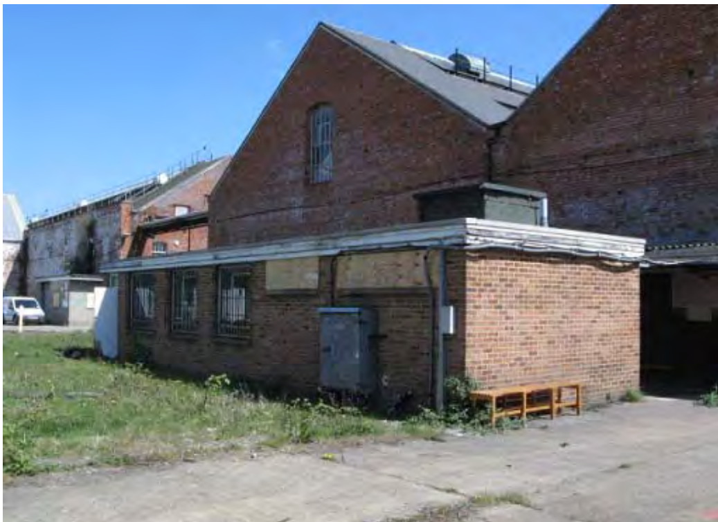
Plate 38. Toilet block (30) looking north with Stores/offices building on right.
