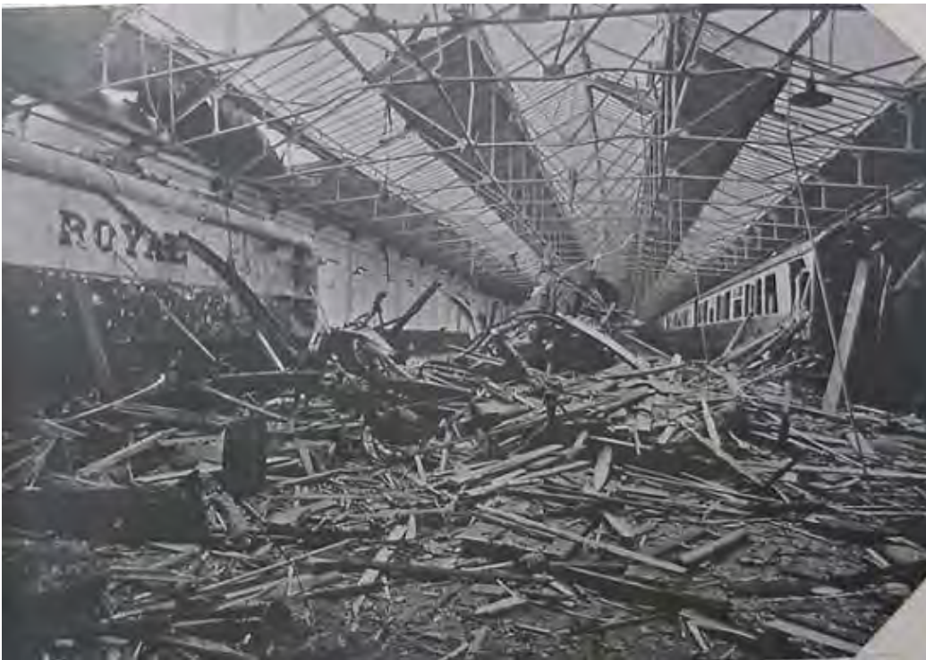
Plate 2. Pullman Shed (22) interior after air raid on 25/10/1940, showing damage to rolling stock and roof trusses.
