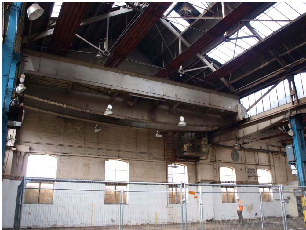
Plate 58. S.H. Heywood & Co Ltd gantry crane, south-east end of Factory former Lifting Shop (15a)
