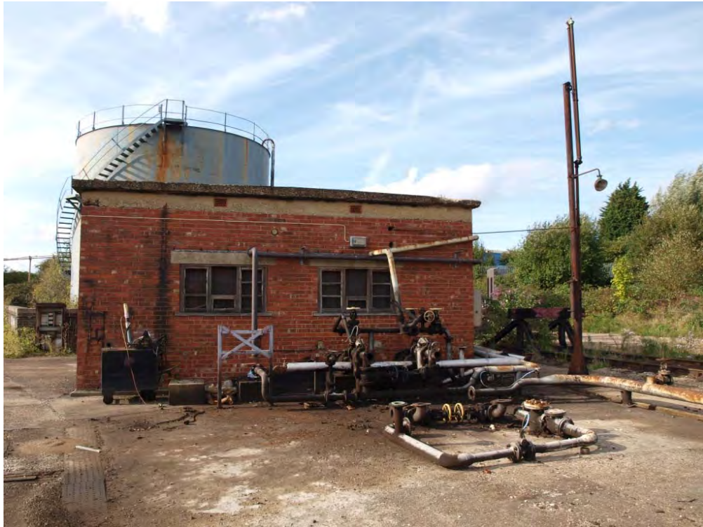
Plate 55. North elevation of Diesel Pump House (6), showing heavy oil/diesel pumps
