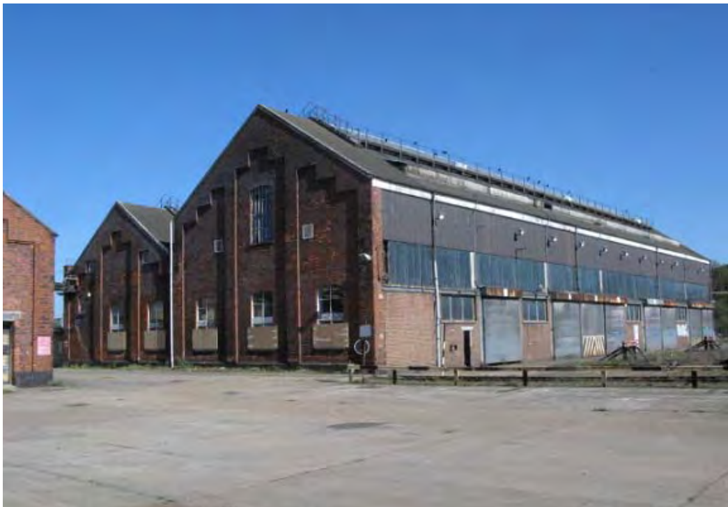
Plate 14. The Factory Maintenance Shed (15a), looking north-west.
