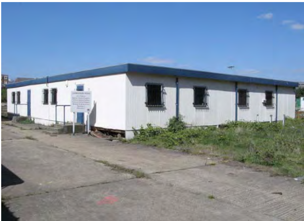
Plate 12. Offices/Portakabins (11 & 18), looking north-west.
