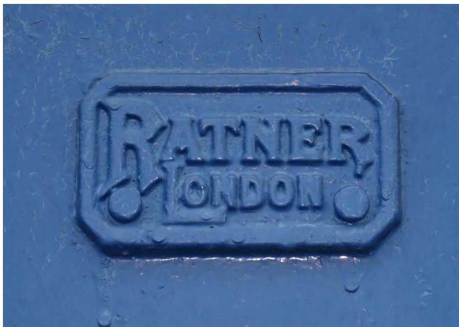
Plate 54. Steel door at west end of Substation B2 (26): detail of maker's nameplate
