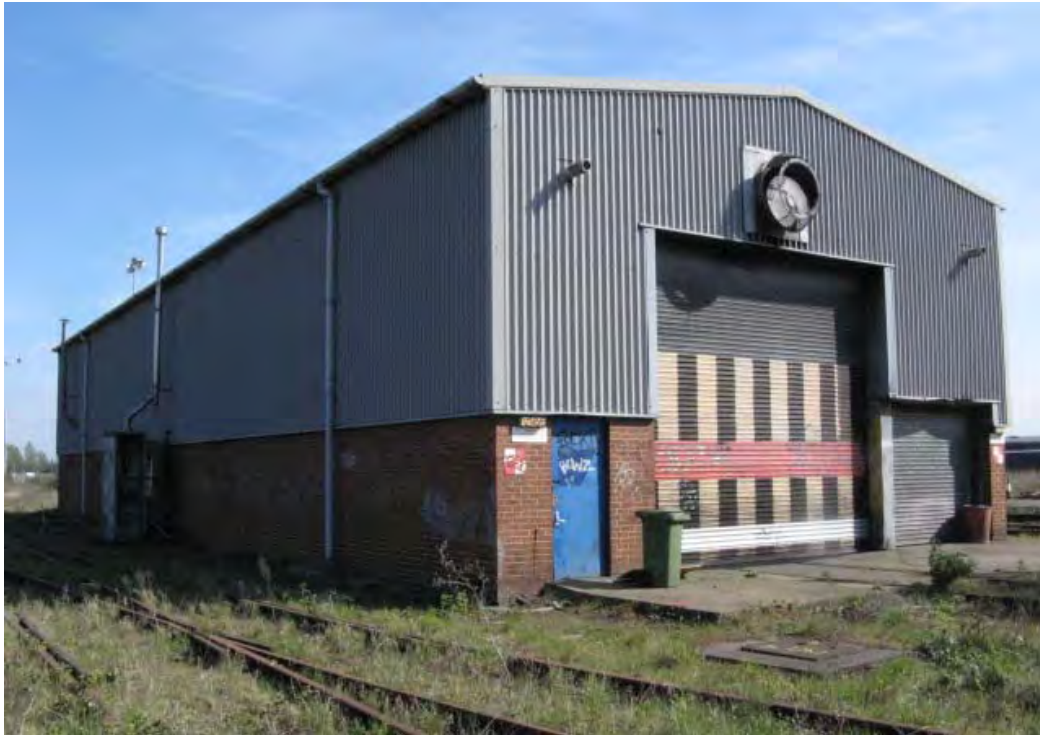
Plate 7. Underframe Cleaning Shed (4).
