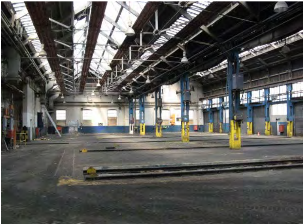
Plate 16. Interior of the Factory Maintenance Shed (15a) looking north-east.
