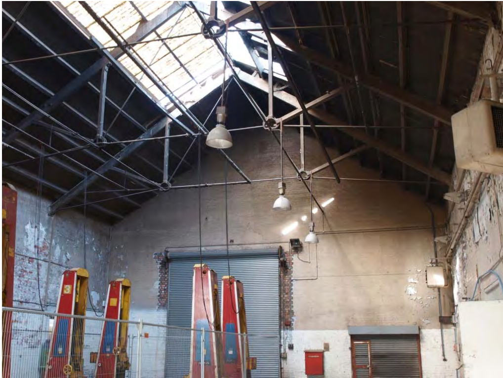
Plate 43. Composite roof truss, Factory former Smiths' Shop (Lifting Bay) (15b).
