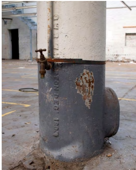
Plate 46. Cast iron column, centre of Stores/Offices building (16a & 16b): detail of manufacturer's stamp
