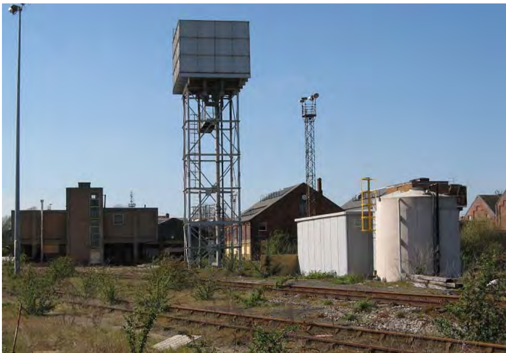
Plate 6. Carriage Washer Treatment Plant (7) and Water Tower (8).
