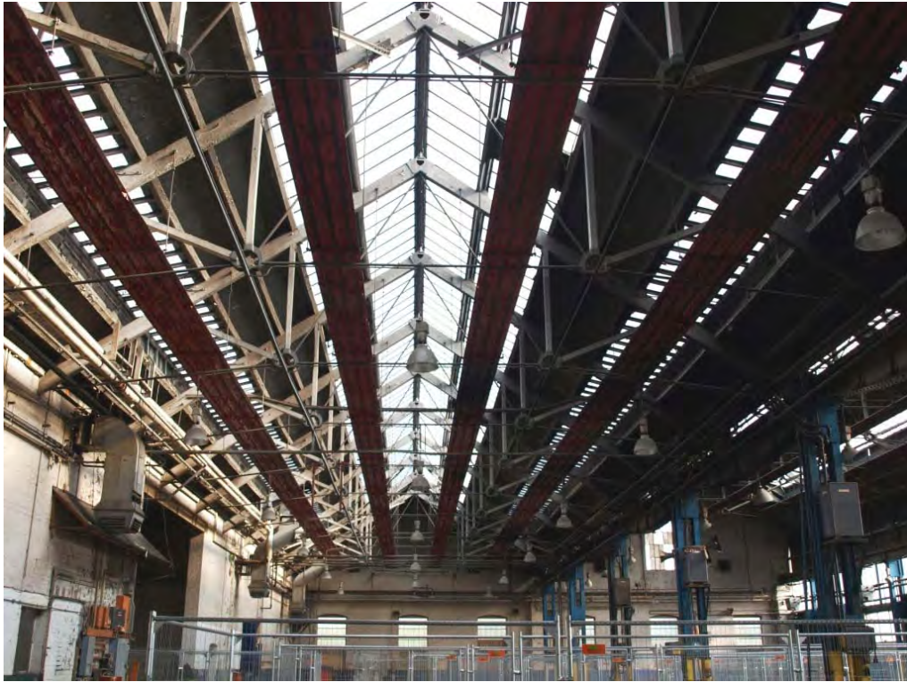
Plate 41. Composite roof truss on west side of Factory (former Lifting Shop) (15a)
