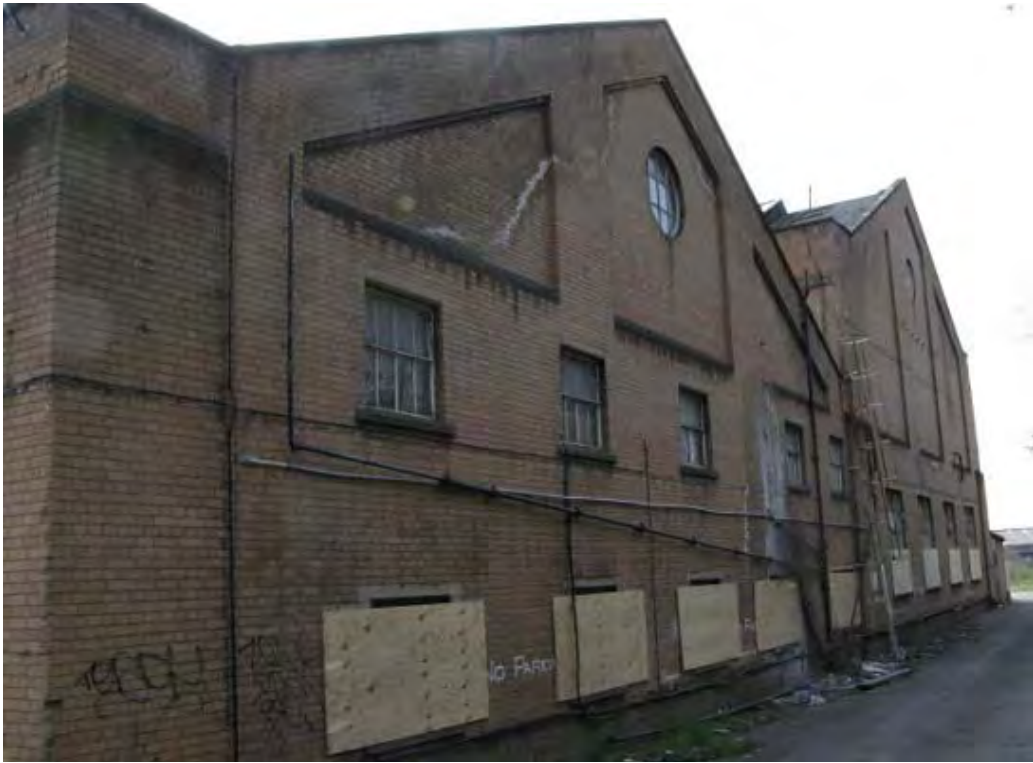
Plate 31. West gable end walls of Pullman Shed (22) on left and Carriage Lifting Shed (23) on right.
