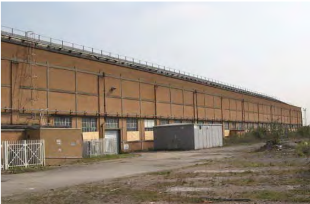
Plate 34. South elevation of Carriage Lifting Shed (23) with SubStation B3 (36) in foreground.
