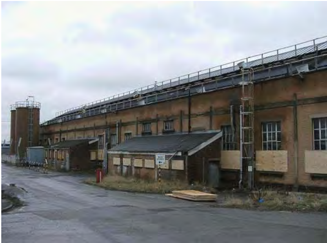
Plate 29. North elevation of the Pullman Shed (22) with Fuel Oil Tanks and grey Pump House (34 & 54) visible on the far left.
