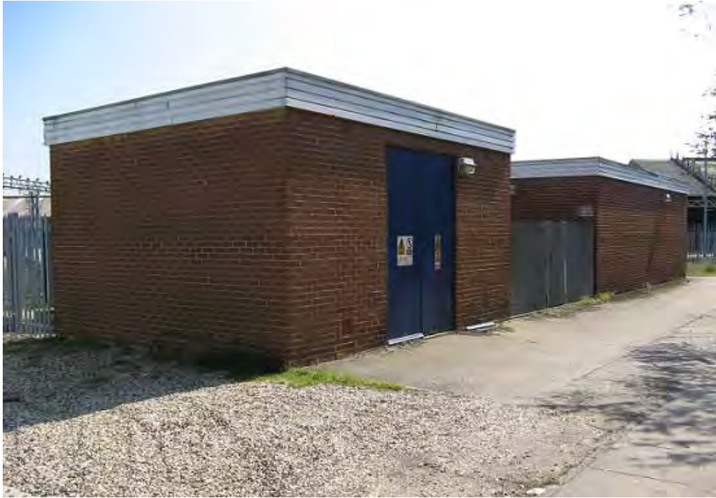
Plate 39. Substation B5 (38) looking south.
