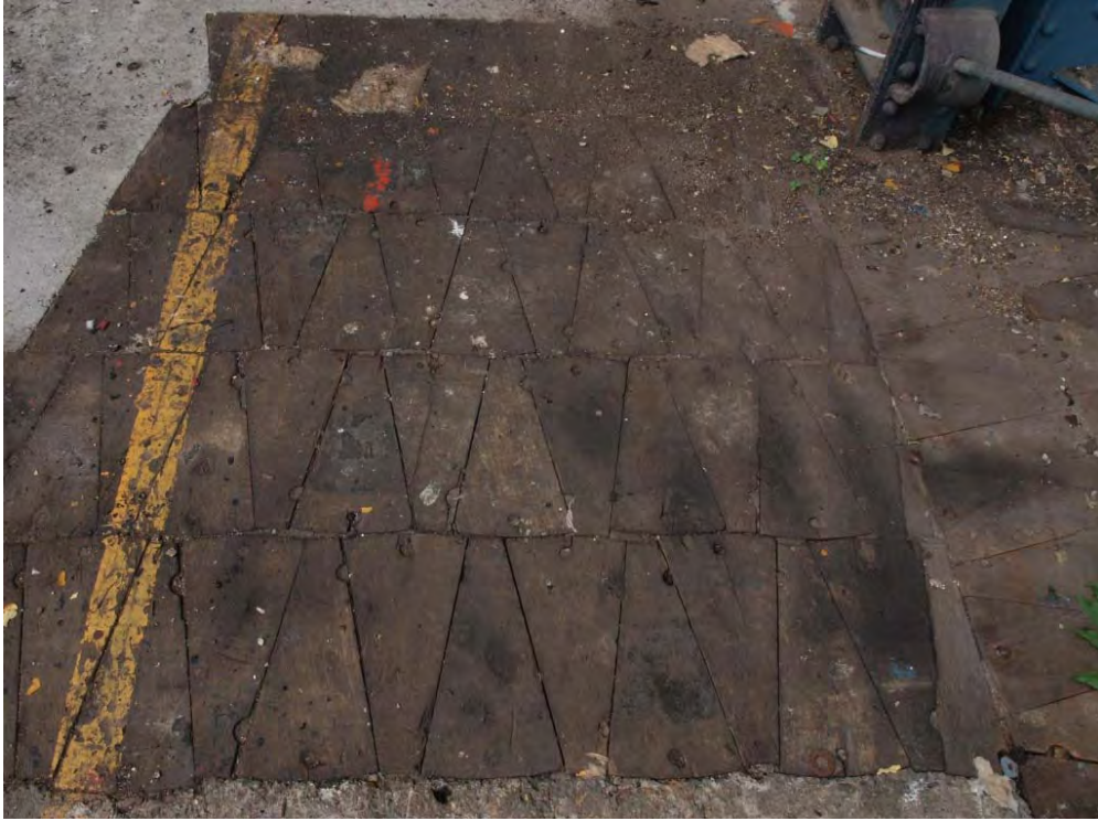
Plate 51. Teak carriage wheel sections reused as flooring in the west end of Carriage Lifting Shop (23)
