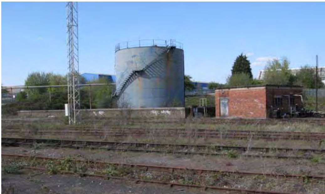
Plate 10. Diesel/Oil Pump House (6) and Bunded Oil Tank (53), looking north-west.
