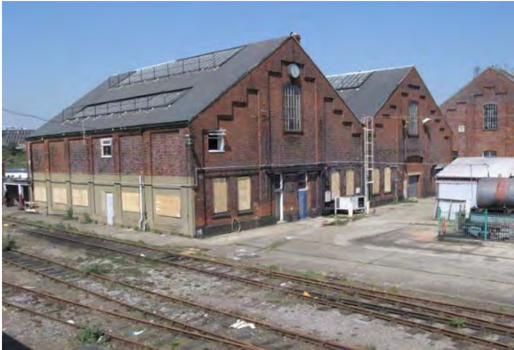
Plate 19. Twin gable end walls of Stores / Offices (16a & 16b), looking north-west.
