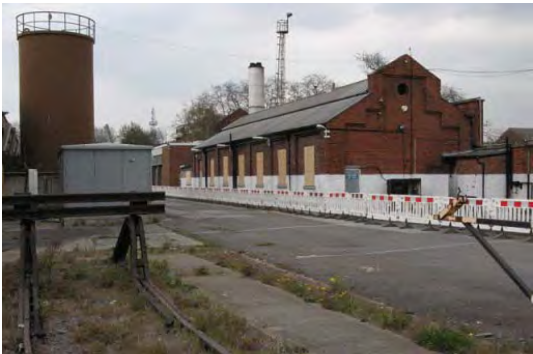
Plate 26. Mess Room/Sand Furnace (20) on right and Fuel Oil Tanks and Pump House (34 & 54) on left.
