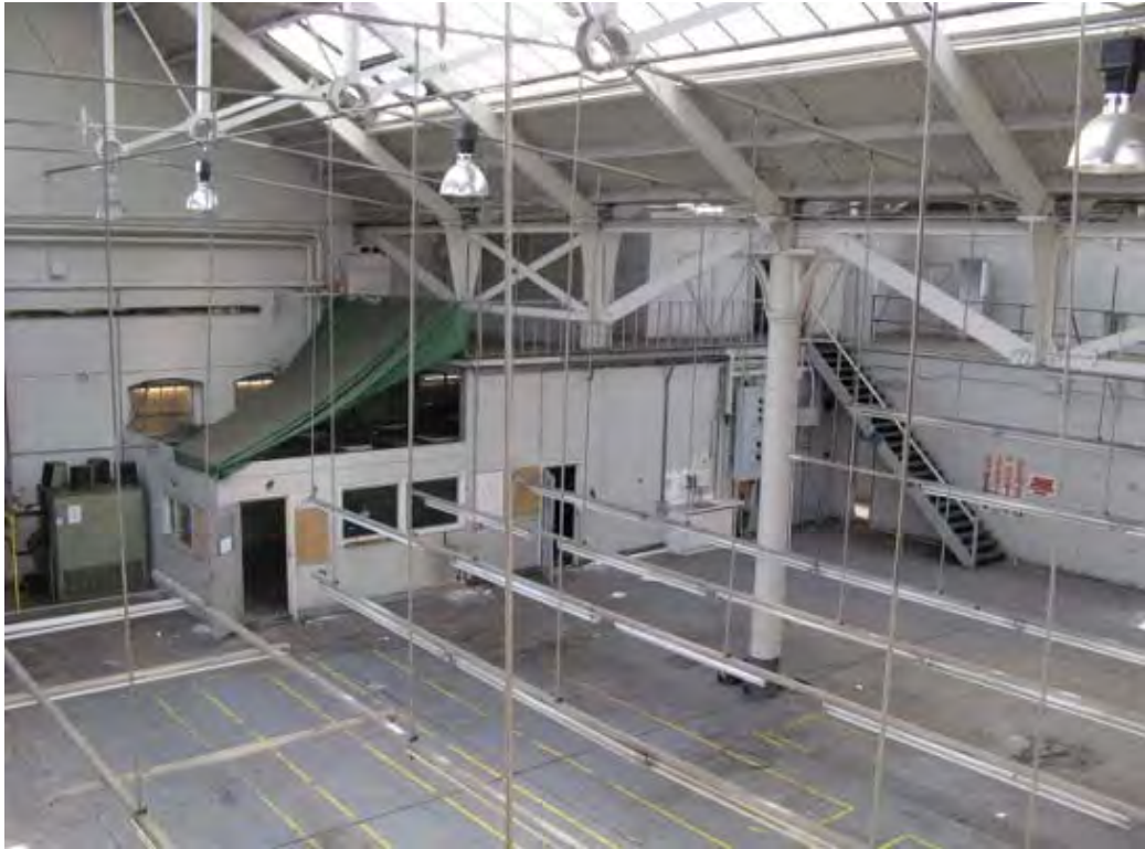
Plate 21. Interior view of Stores/Offices (16a & 16b), looking south-east across central open area to ground floor offices against east and south walls.
