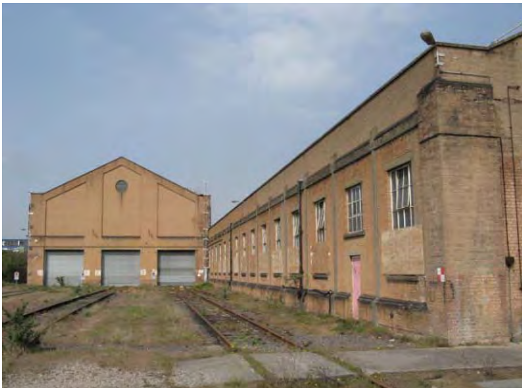
Plate 30. South elevation of Pullman Shed (22) with east gable end wall of Carriage Lifting Shed (23).
