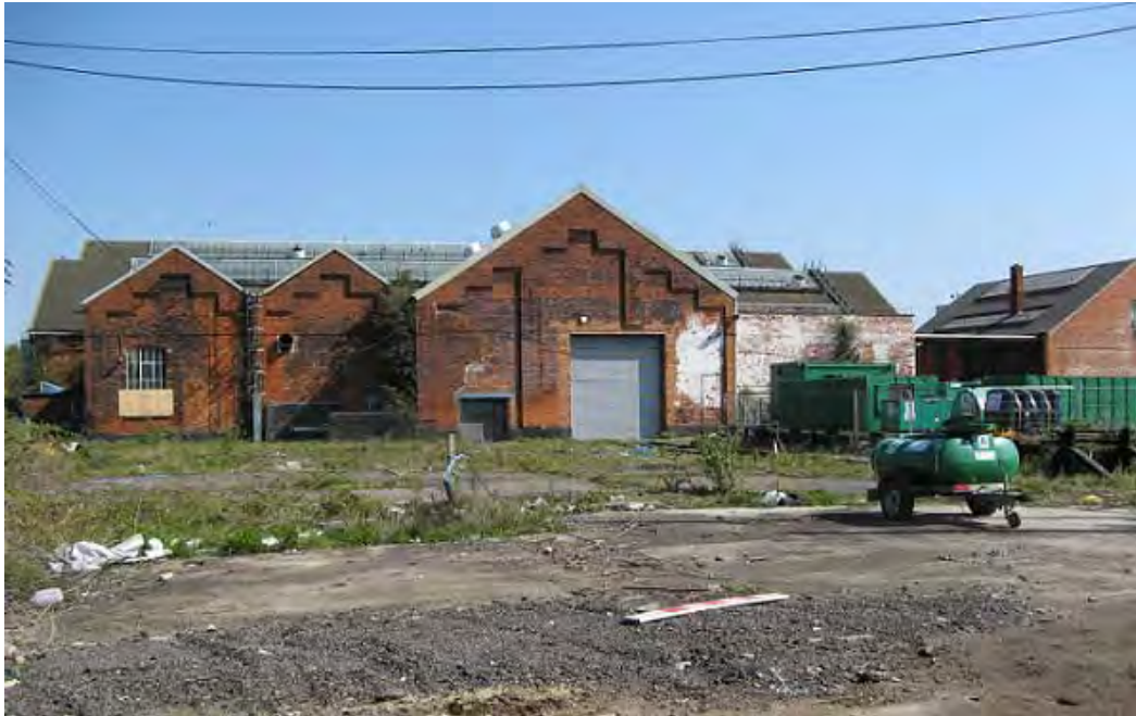
Plate 15. South elevations of The Factory, central gable end wall of Lifting Bay (15b) and two gable end walls of Boiler House on left (15c).
