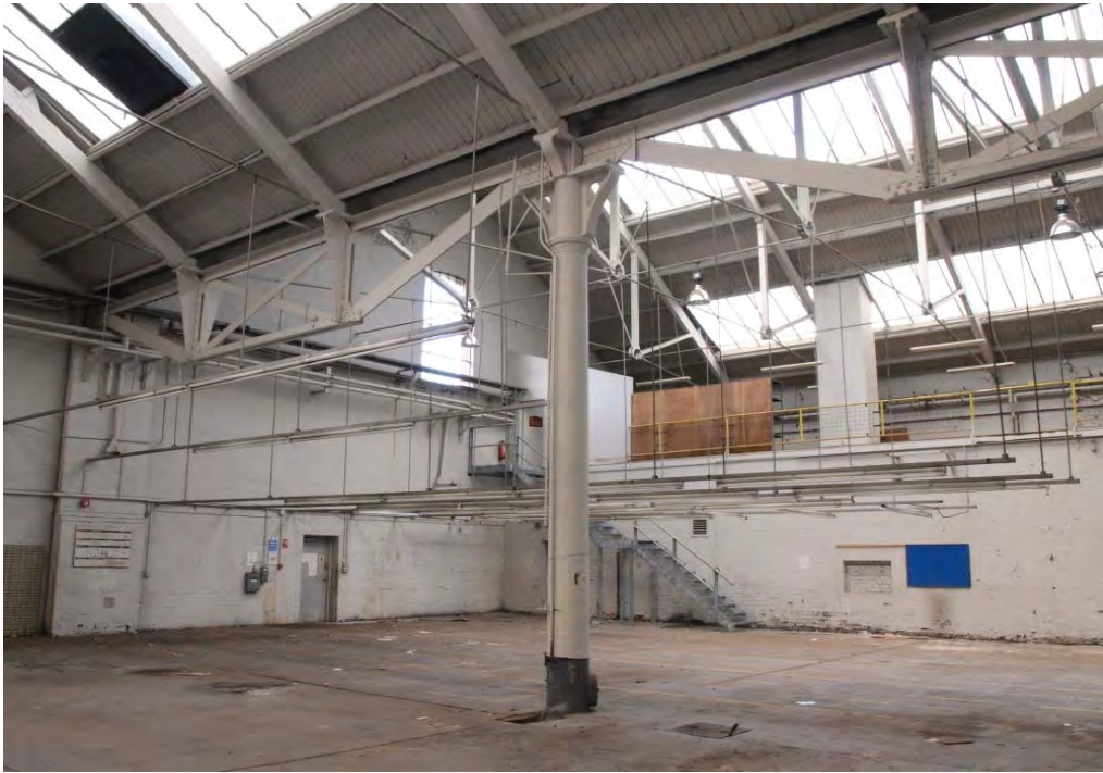
Plate 47. Cast iron column, centre of Stores/Offices building (16a & 16b)
