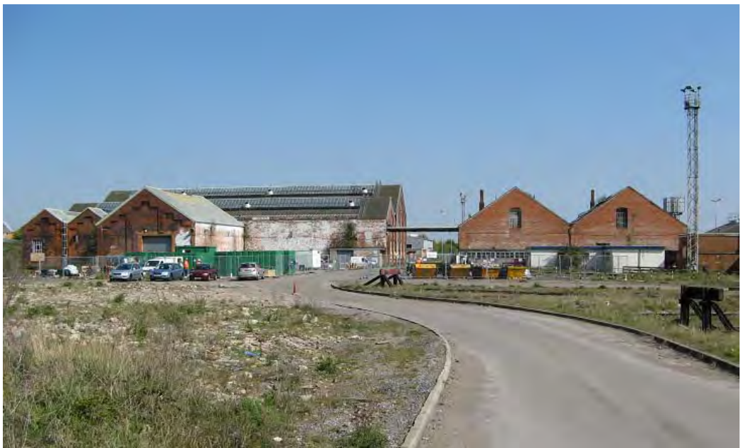
Plate 20. Gable end walls of west elevation of Stores/Offices (16a & 16b) on right with the Factory (15a, 15b & 15c) on left. The surviving turntable (28) is just out of sight on the right and the foreground is part of the area covered by the original 1905 Engine Shed.
