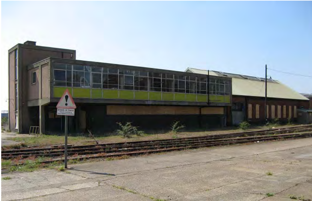
Plate 23. Amenity Buildings (17b & 17a), looking south-west.
