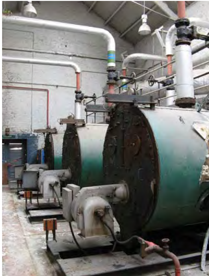
Plate 18. Interior of the Factory Boiler House (15c), looking west.
