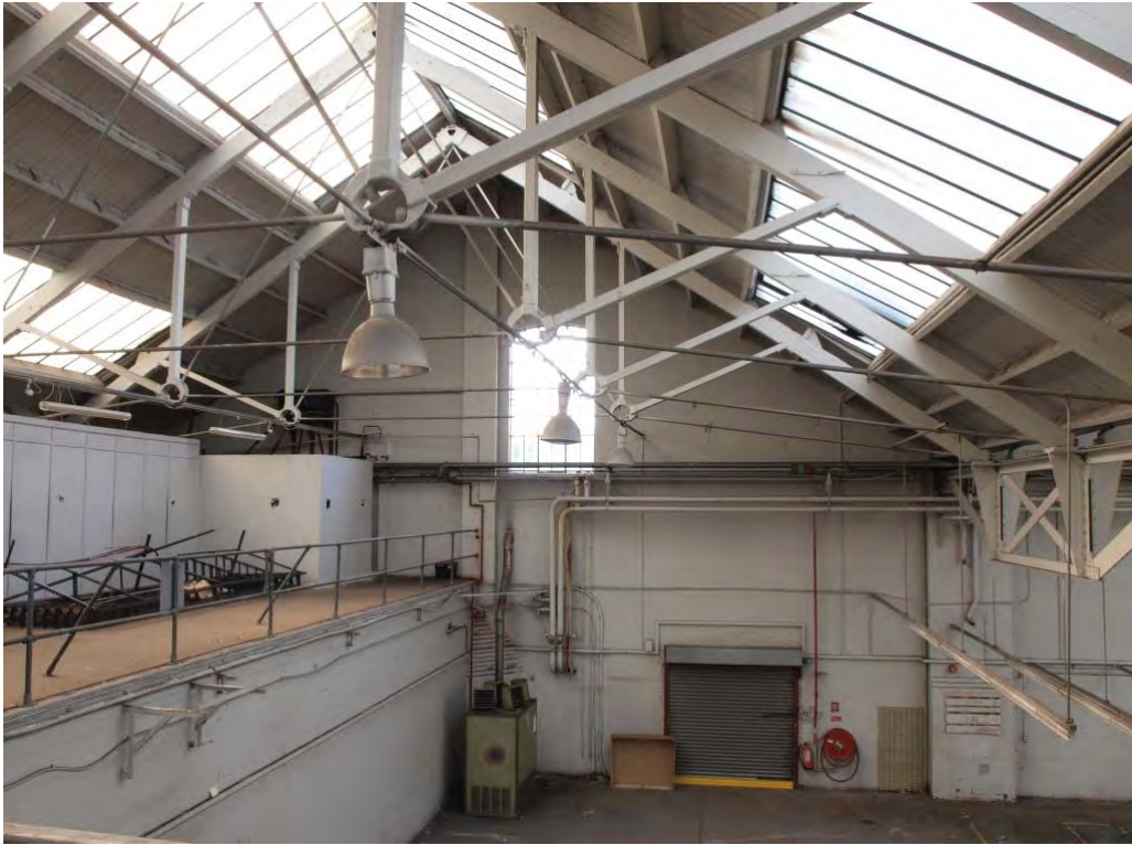
Plate 49. Composite roof truss, south side of Stores/Offices building (16a & 16b)
