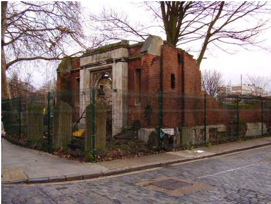
Figure 9. View of ruined Baptist Church, from Stepney Green
