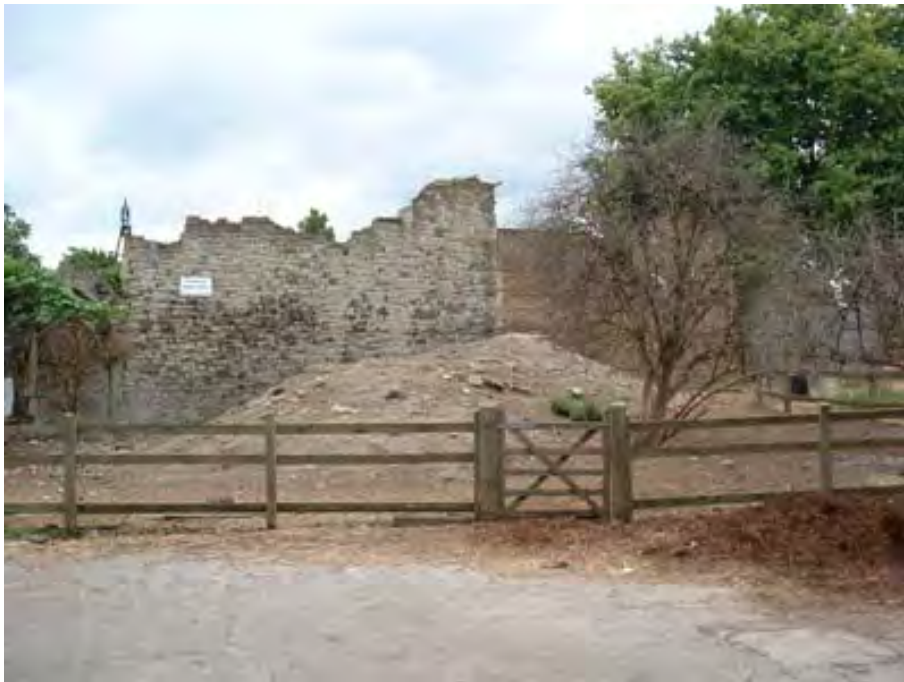
Figure 6. View of the rear wall of the Congregational Church from the north
