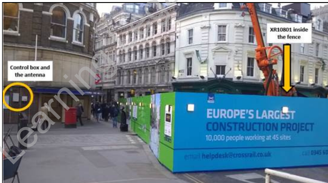
Figure 4- C502 site hoarding impeding XR10801
