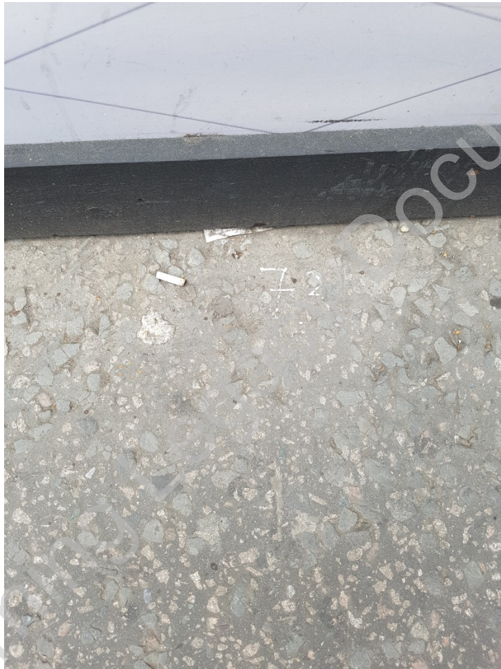
Figure 5- LP12173B Location on Pavement
