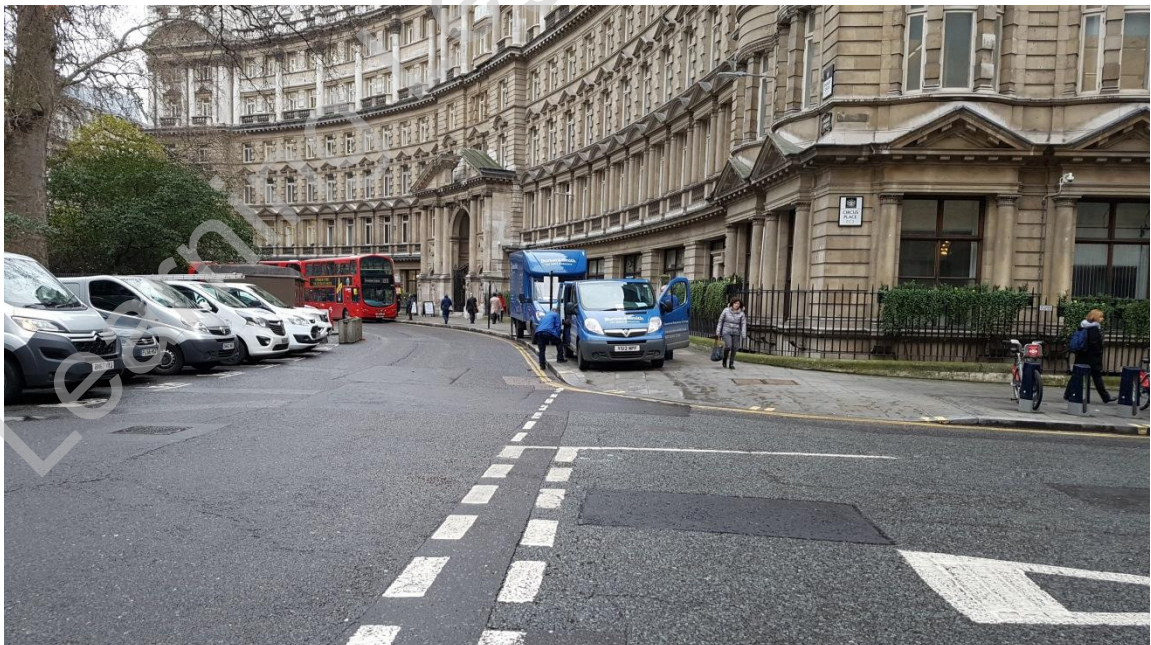
Figure 5. Finsbury Circus pavement, 23-25 London Wall - HGV parked over the studs
