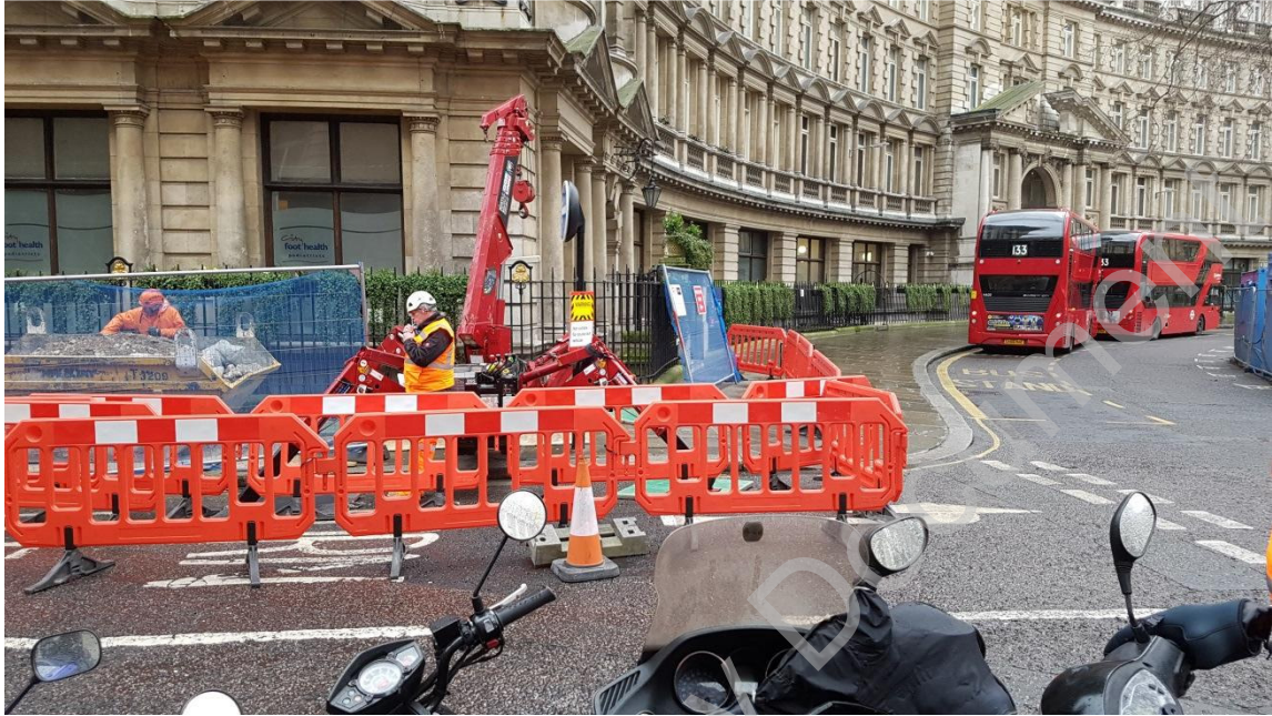
Figure 6. London Wall basement works
